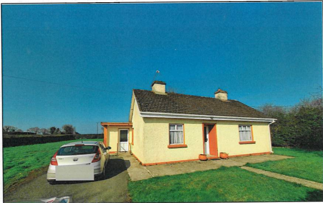
Photo 1: Front elevation of existing dwelling
