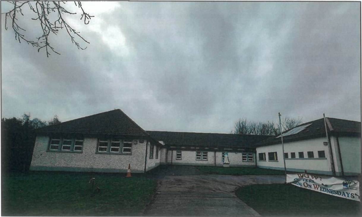
Photo 1: Front (north) elevation of subject site
