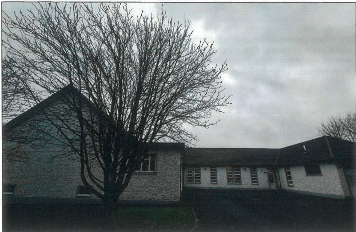
Photo 2: Side (west) elevation of the subject site
