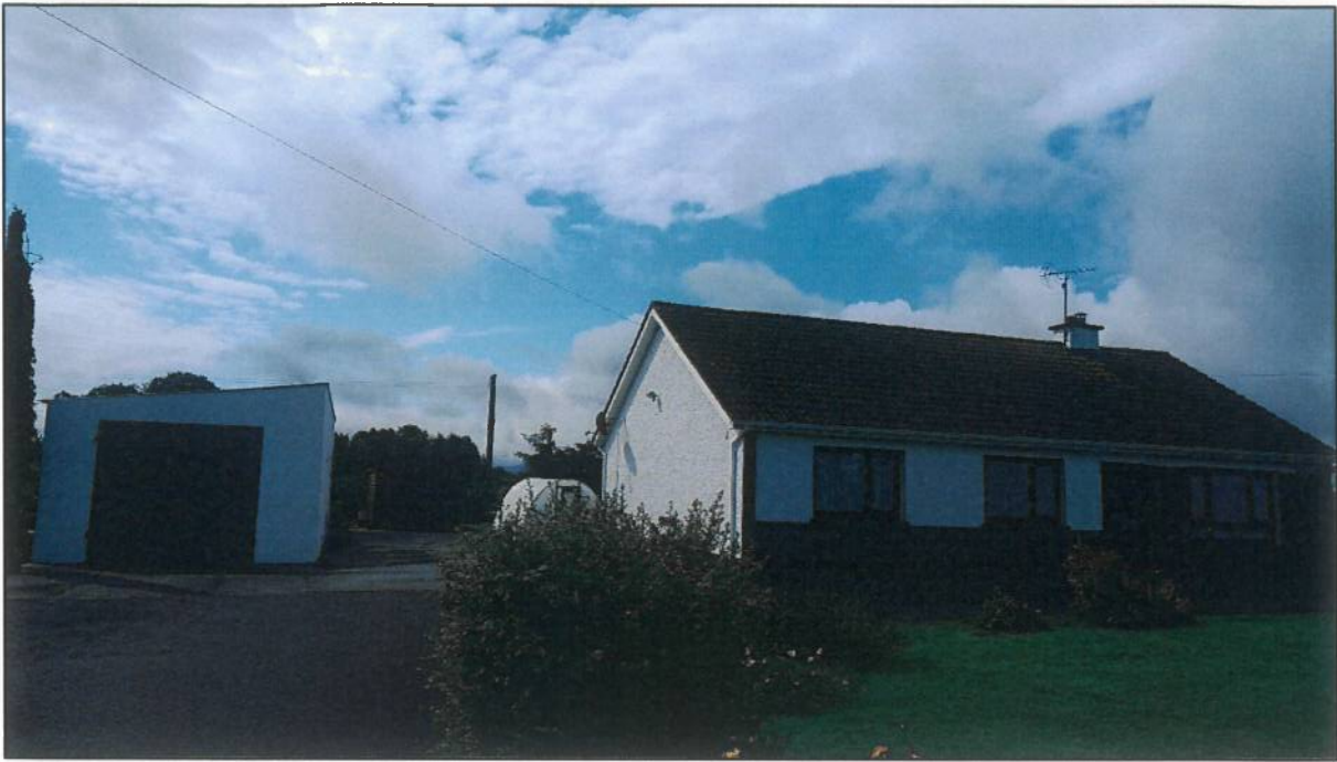
Photo 1: Front elevation of existing dwelling
