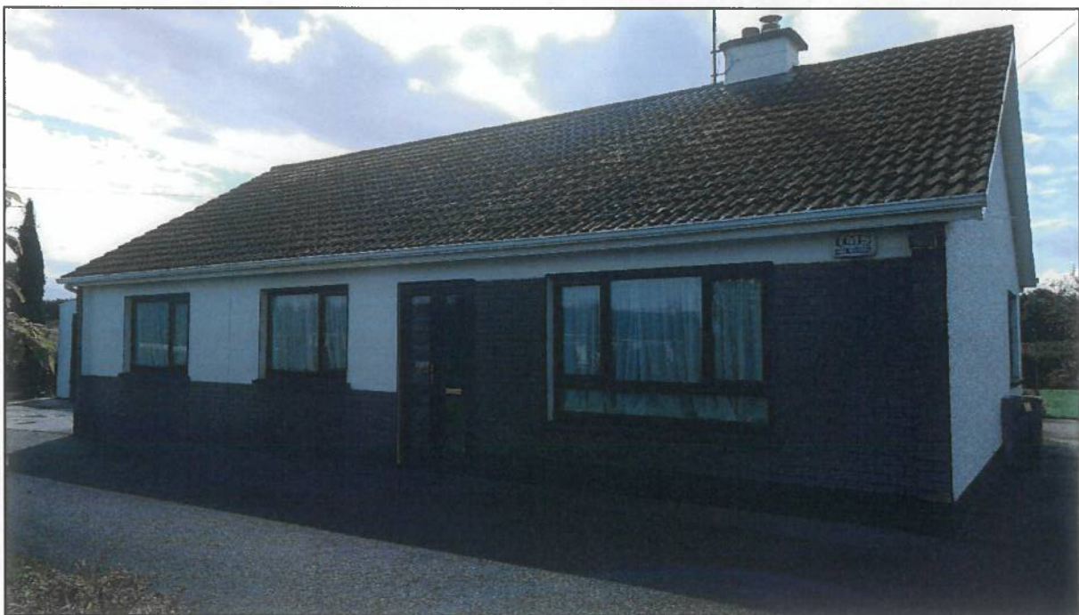
Photo 2: Front elevation of existing dwelling
