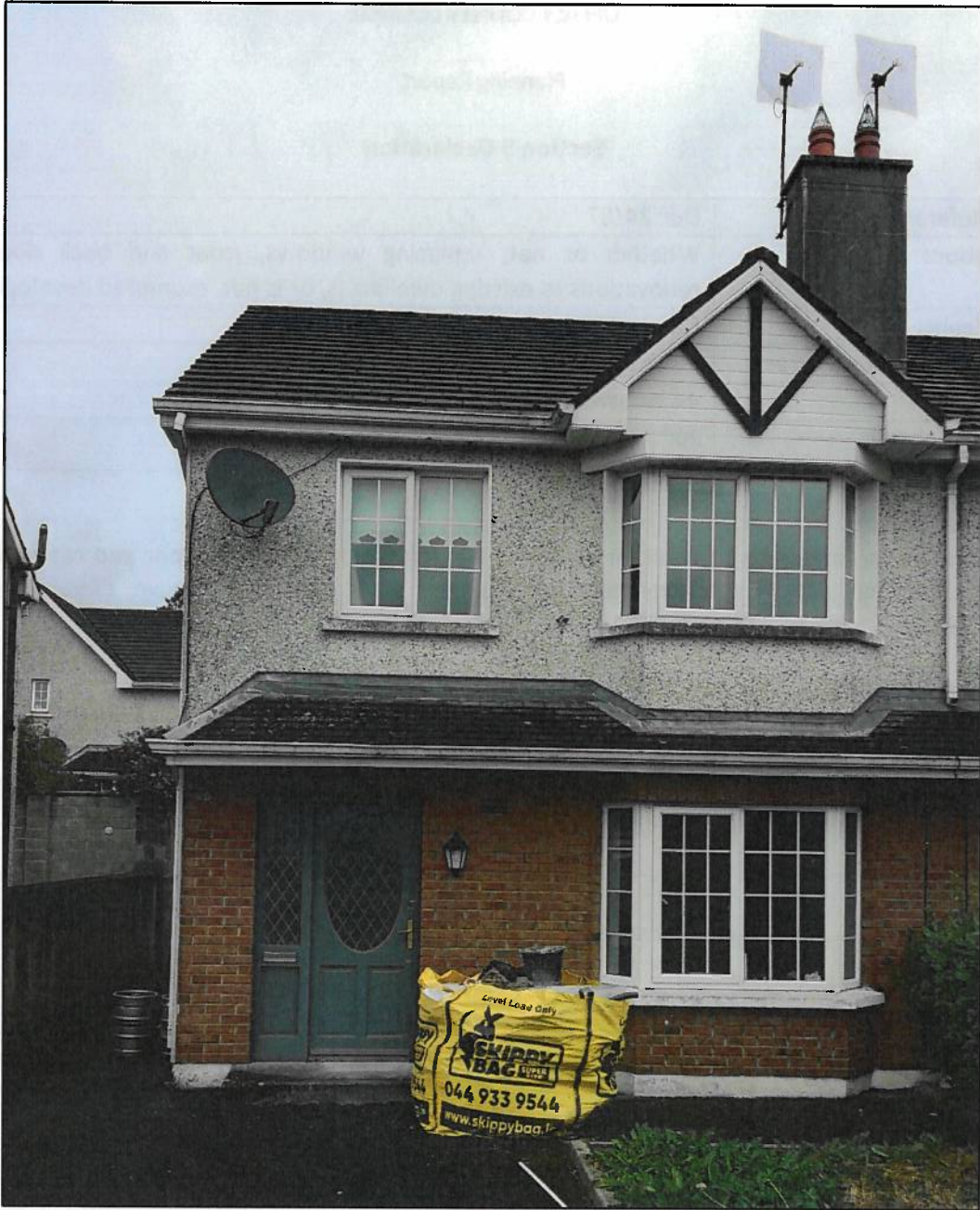
Photo 1: Front (south) elevation of existing dwelling
