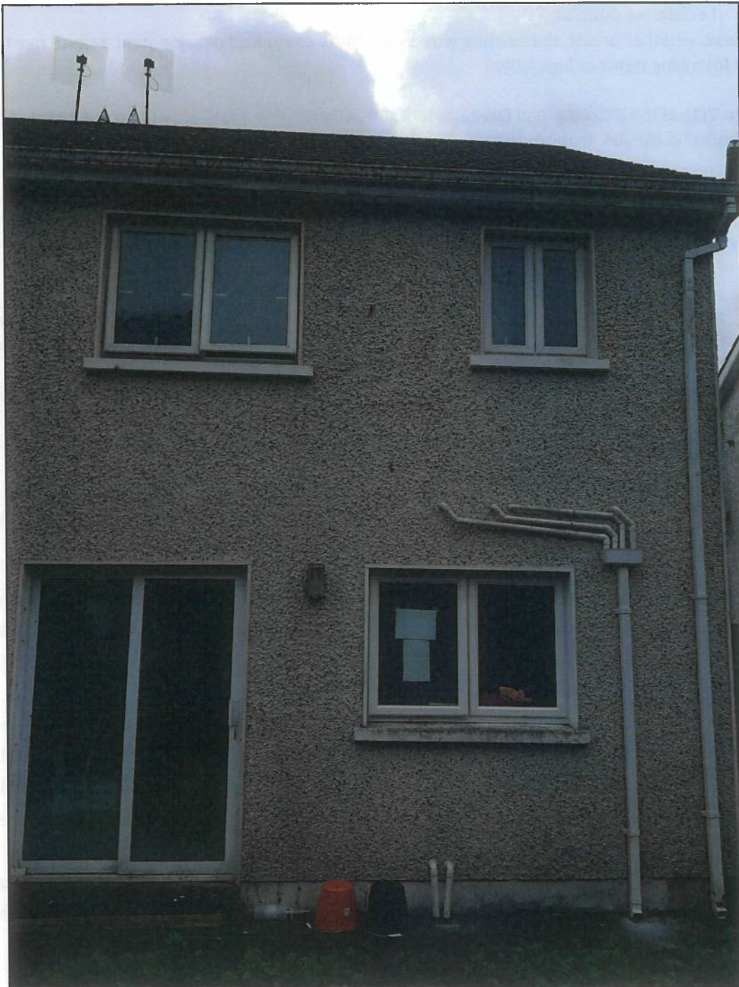
Photo 2: Rear (north) elevation of existing dwelling
