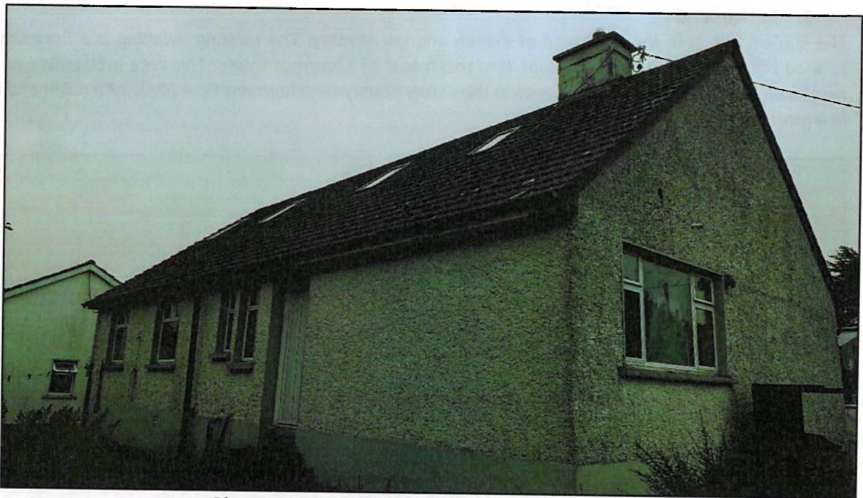
Photo 2: Rear (west) elevation of existing dwelling
