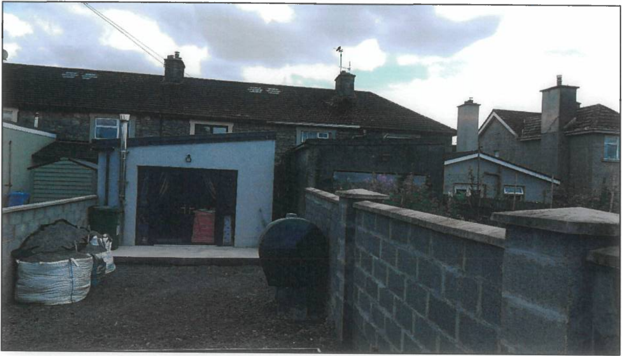
Photo 1: South-east view of rear extension
