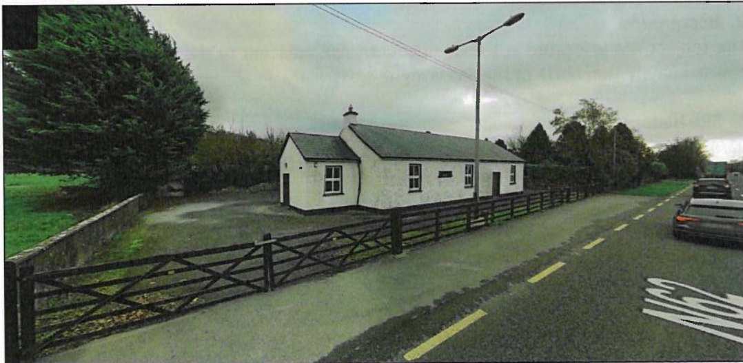
Photo 1 – Subject Site (Google image – November 2022).
