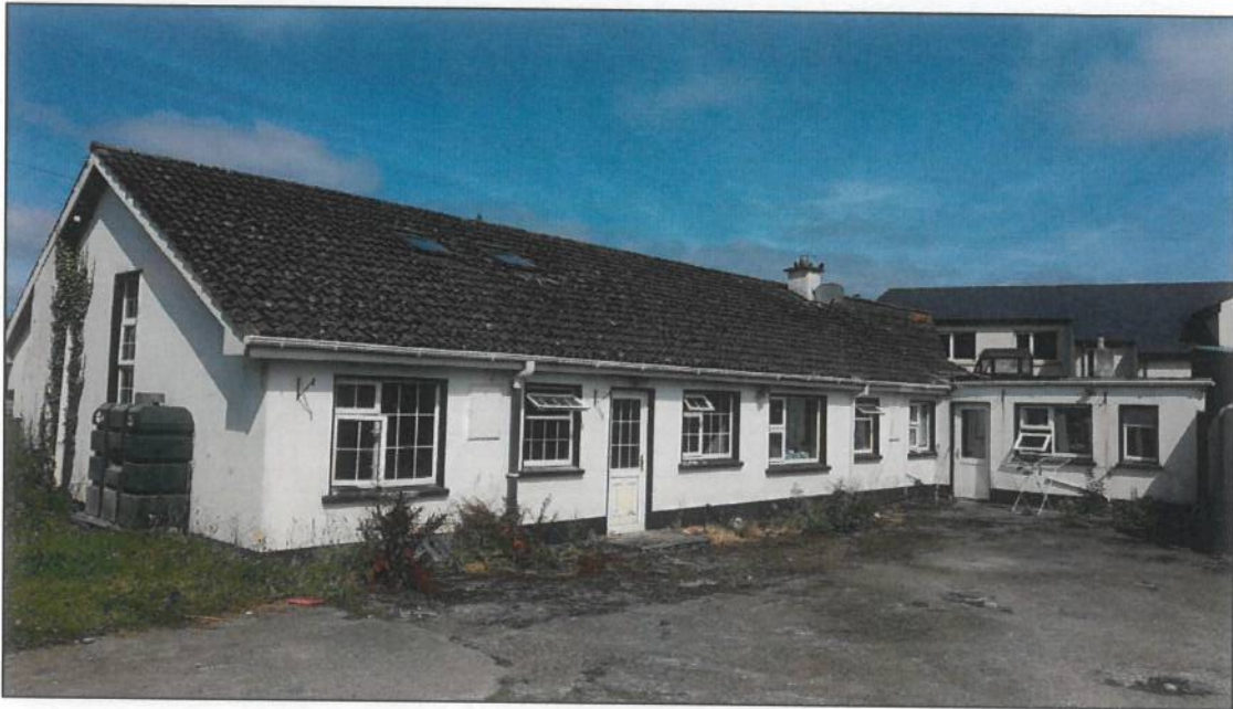
Photo 2: Photo of rear exterior of 2 Barnagrotty Road.
