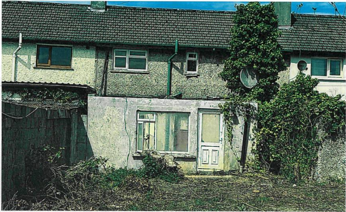
Fig 1: Photograph showing the rear of the dwelling which indicates an existing extension.
