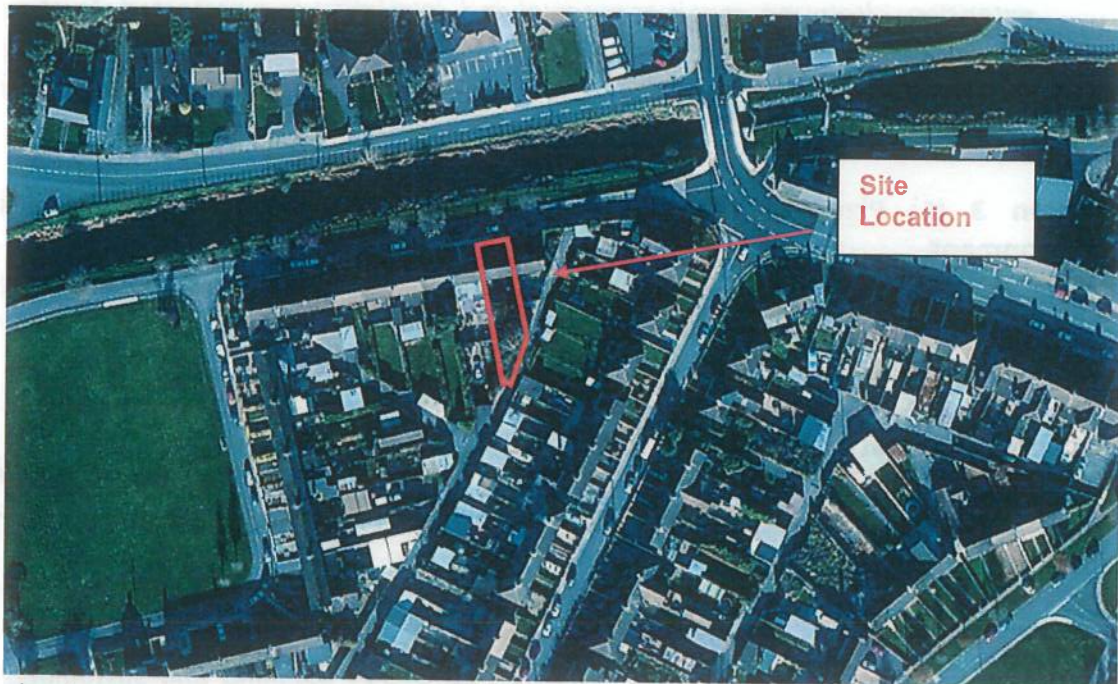
Figs 4: Aerial image of location of site
