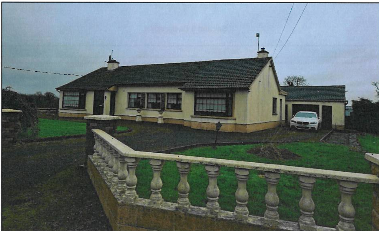
Photo 1: Front (east) elevation of existing dwelling
