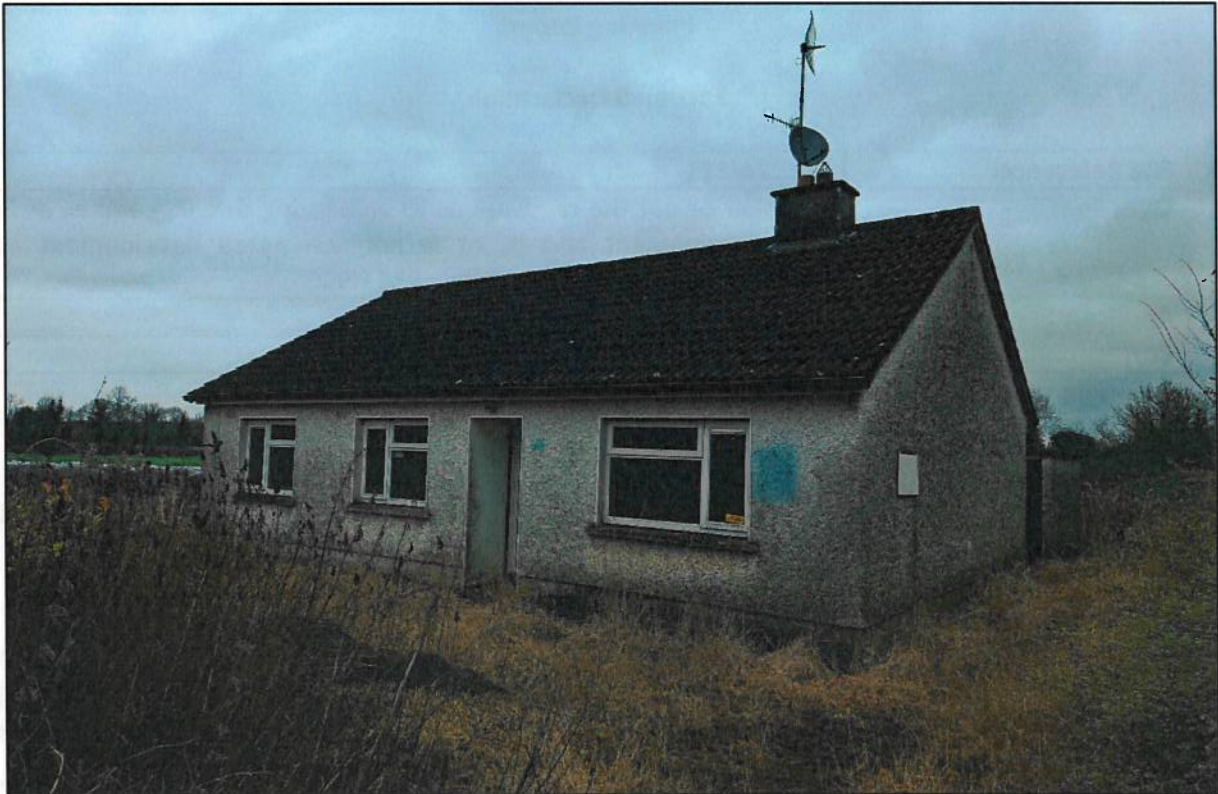
Photo 1: Front (south) elevation of existing dwelling
