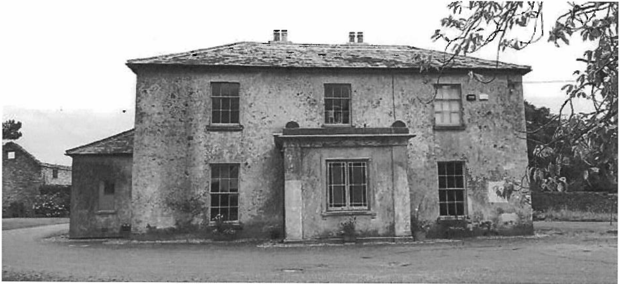
Front elevation – note connections at first floor level (to be removed with underground works)
