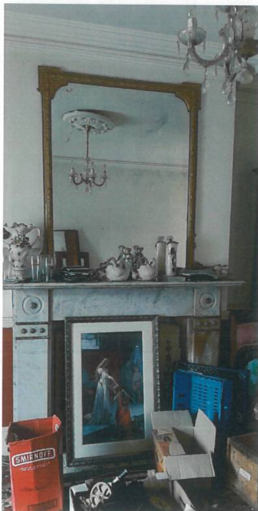
Some decorative features remaining including chimneypieces to former bedrooms and upper living room with overmantle and moulded cornice. Excellent upper windows with architraves, shutters and timber paneling.
