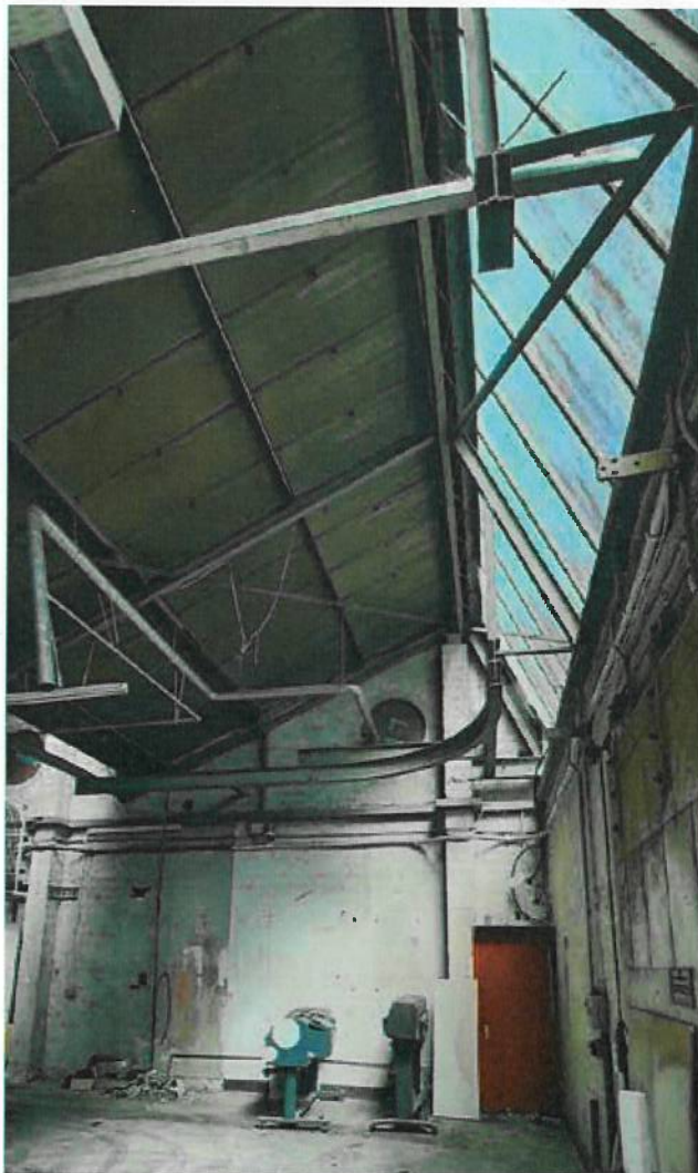
Interior, vast sawtooth structure with asbestos roof
