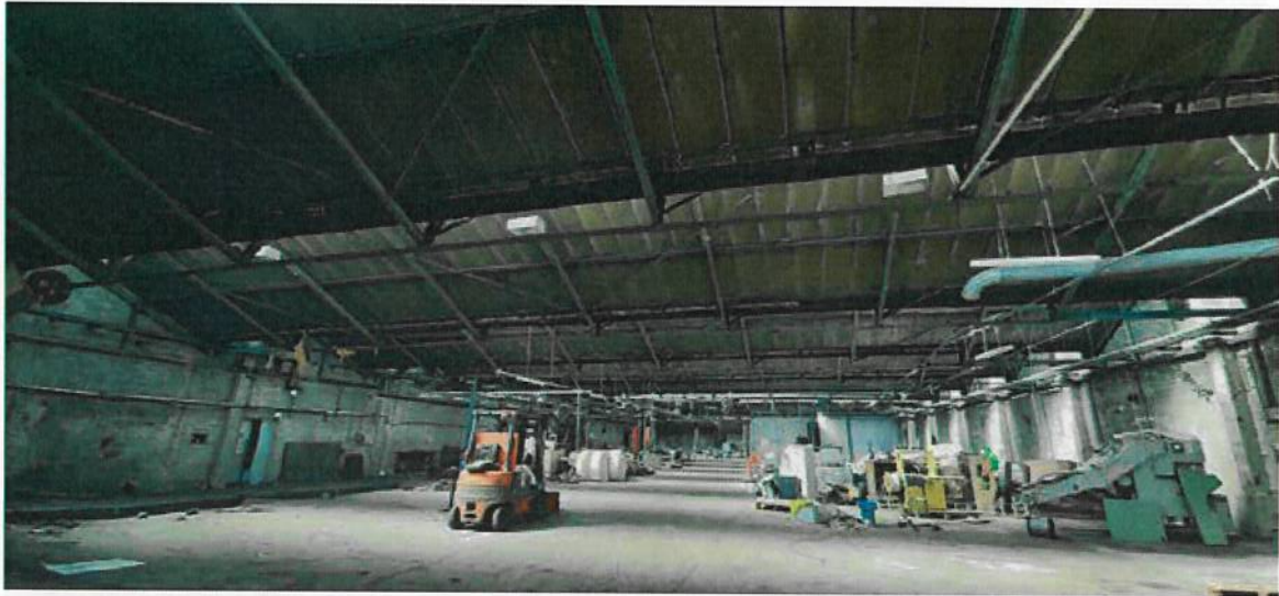
Interior, vast sawtooth structure with asbestos roof
