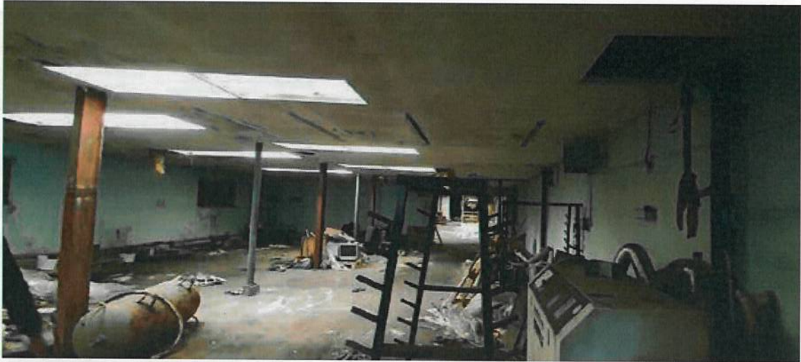
Internal view of flat roofed building with asbestos roof built beside sawtooth building
