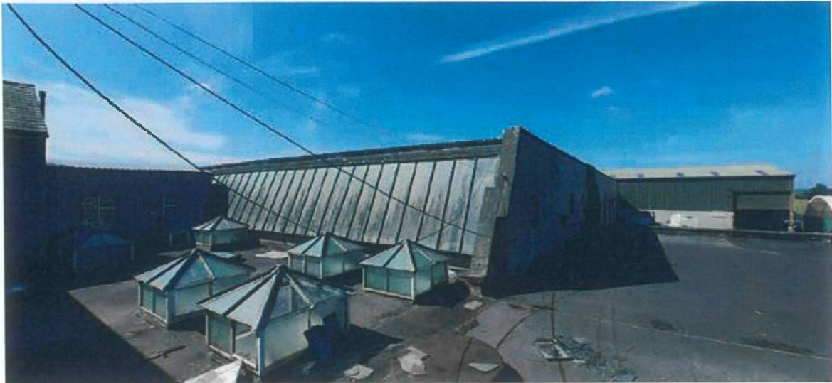
Sawtooth roof viewed from first floor of main building
