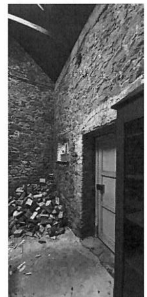
Coach house GF RHS - 20220411_112700.jpg
