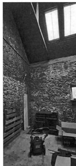
Coach house GF RHS - 20220411_112657.jpg
