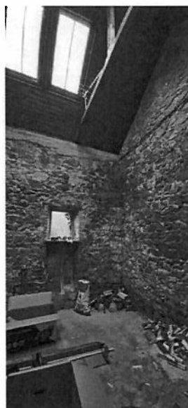
Coach house GF RHS - 20220411_112655.jpg
