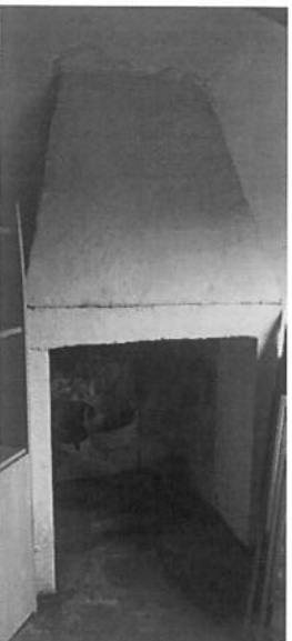
Boiler house fireplace - 20220411_110151.jpg
