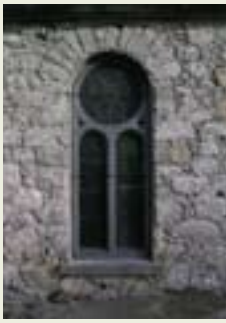
PLATE 30. Nave south window
