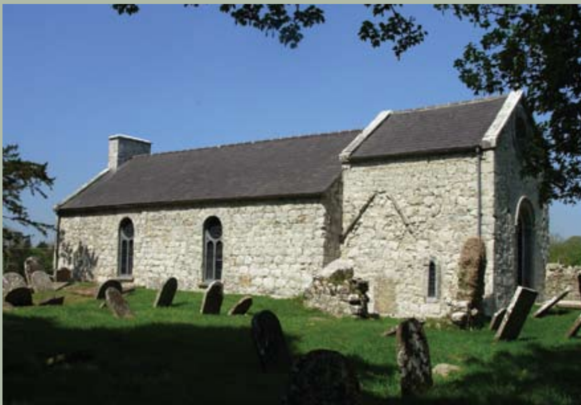
PLATE 22. External face of south wall of the nave and chancel church with roofline of south porticus visible.
