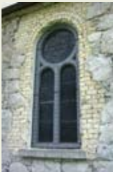
PLATE 31. Nave south window
