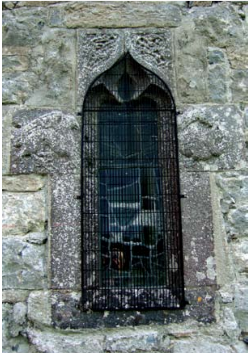
PLATE 5. 15th century single light ogee-headed window in north wall of nave.
