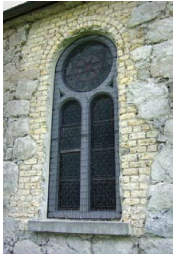
PLATE 8. 19th century brick window inserted into north wall of nave.
