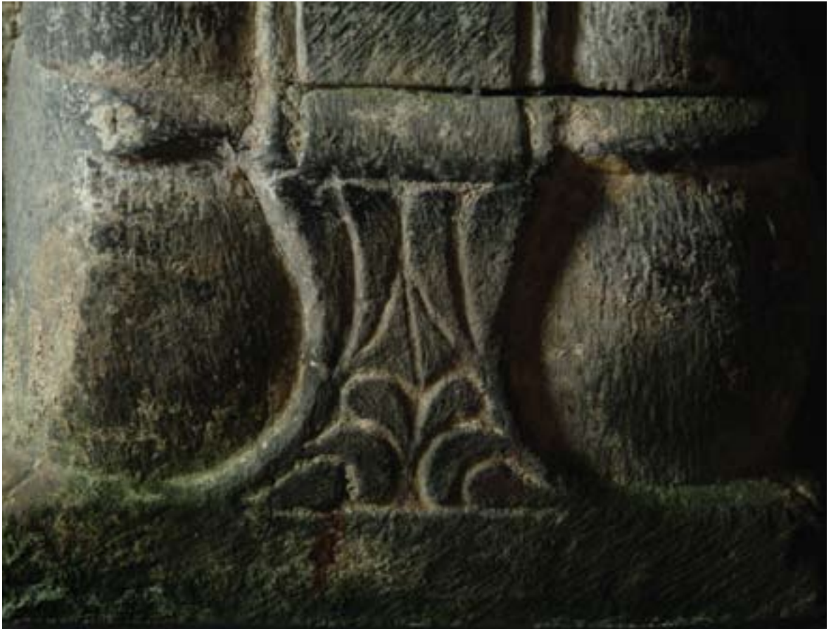
PLATE 47. Bulbous bases of engaged columns and decorative floral motif of the chancel arch. The floral motif is only found on the base of the north side of the chancel arch.
