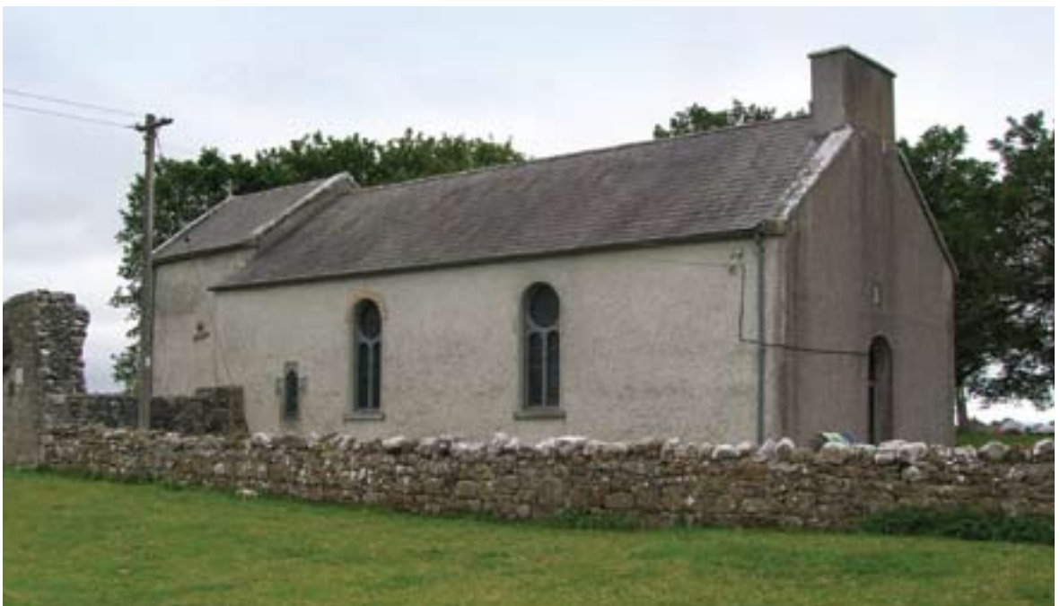
PLATE 2. Northwest face of Rahan Church prior to conservation.
