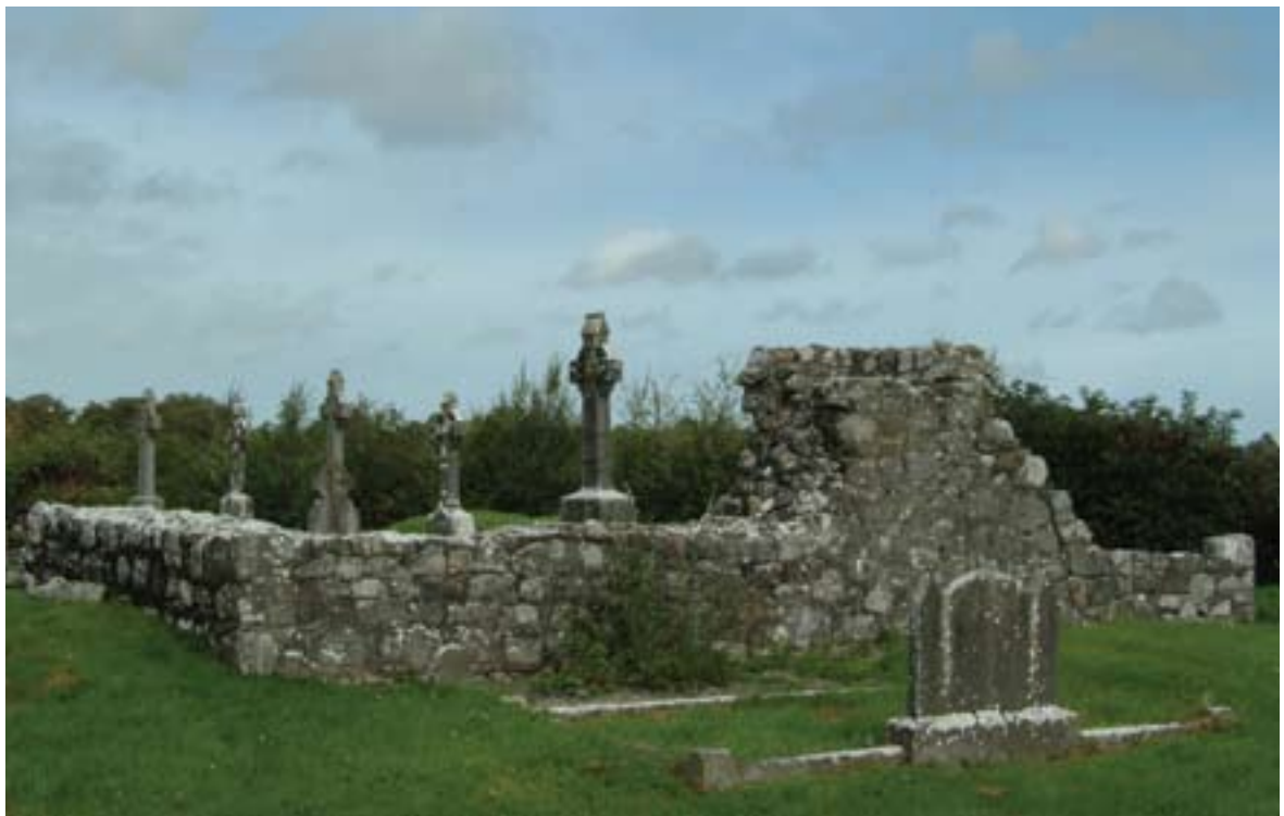
PLATE 37. Remains of possible tower house in modern Roman Catholic cemetery.
