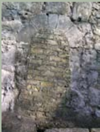
PLATE 23. South face of bricked up doorway leading from chancel into south porticus.
