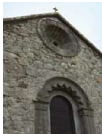
PLATE 21. External face of east gable showing round Romanesque window and 20th century window inserted by William Martin.
