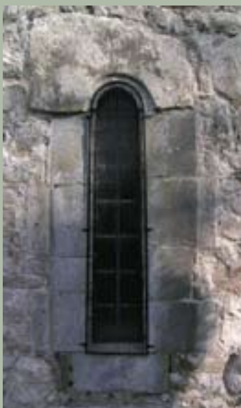
PLATE 24. Single light round headed window in south wall of chancel.
