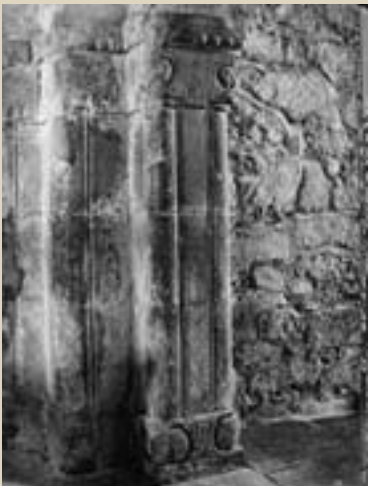
PLATE 16. View of internal face of the engaged columns on the north side of the chancel arch (Henry 1970).
