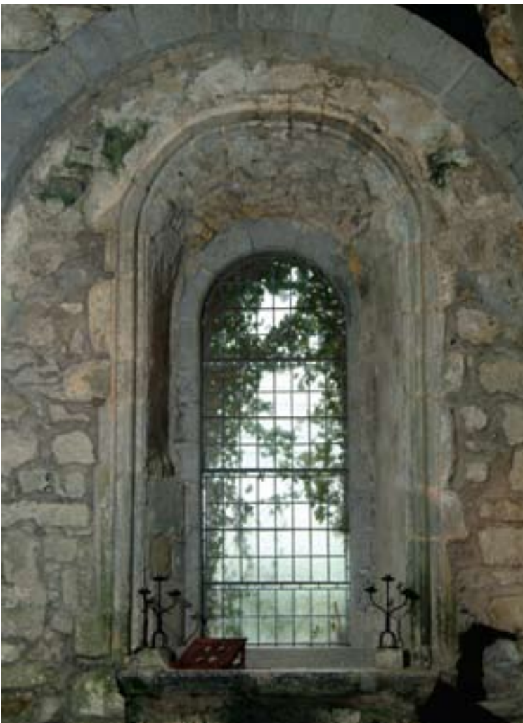
PLATE 20. Internal face of 13th century east window.
