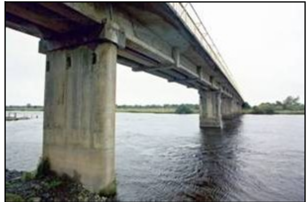
Fig 3.32a (left): A simple metal girder Bord na Mona railway bridge over Silver River, Stonestown Td (023-021). Fig 3.32b (right): Garryduff Bridge, a multi-beam concrete bridge over the Shannon at Shannonbridge (013-018).
