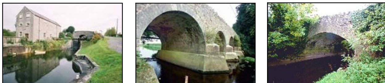
Fig 4.2a (left): This store, bridge and quay form a pleasing combination at the 33 rd lock on the Grand Canal, Ballingowan Glebe Td (014-032). Fig 4.2b (middle): Millbrook Bridge is a striking landscape feature over the Figile River (027-003). Fig 4.2c (right): Road bridge over Blackwater at Clonever Td – a rare example of a concrete block arch, in this case a 1920s rebuild (013-015).
