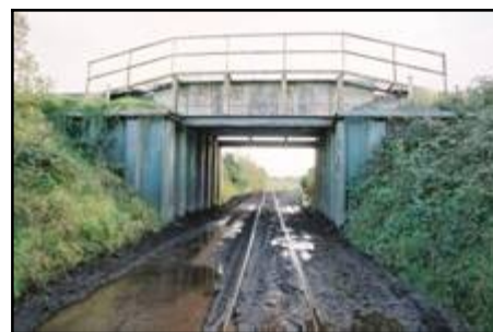
Fig 3.36 Mainline railway bridge over peat railway at Bellair (007-023).
