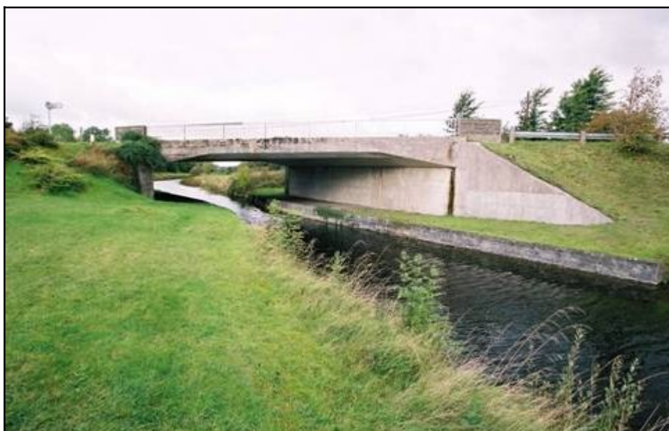
Fig 5.6 Noggus Bridge, a late 1900s replacement skew road bridge over the Grand Canal (014-023).
