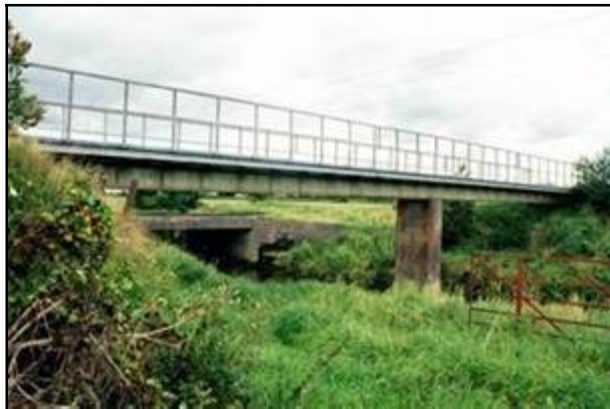
Fig 3.32a (left): A simple metal girder Bord na Mona railway bridge over Silver River, Stonestown Td (023-021). Fig 3.32b (right): Garryduff Bridge, a multi-beam concrete bridge over the Shannon at Shannonbridge (013-018).
