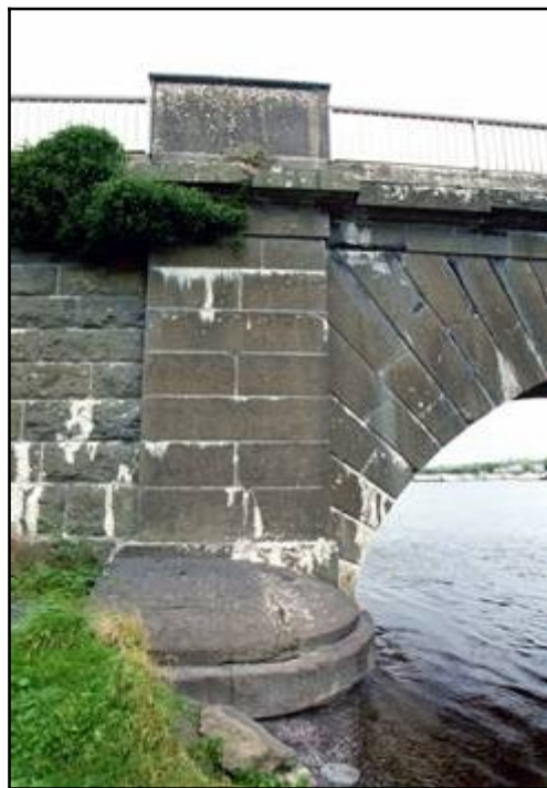
Fig 3.14 Left : Ashlar stonework on Banagher Bridge (021-006). Above : Plaque recording the bridge's construction between 1841 and 1843.
