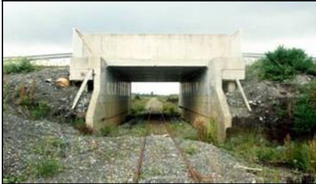
Fig 2.18a ( top left ): Kilcolgan Bridge, a beam and slab structure of c.1951 over Brosna (015-006). Fig 2.18b ( top right ): Pre-cast beam and slab bridge of 2002 over Dublin-Galway railway, Cloncoher Td (025-016). Figs 2.19c and 19d ( bottom ): This pre-cast concrete box-section bridge of 1999 carries the Daingean-Tullamore road over a Bord na Mona railway (018-041). The individual units are tied together with metal rods.
