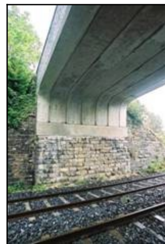
Fig 3.37 Replacement inverted U-beam deck on road bridge, Ard Td (026-005).
