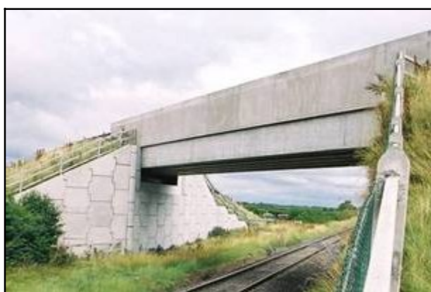
Fig 3.38a (left): Accommodation bridge at Clonyquin Td; note pre-cast concrete units on abutments and side walls (033-015). Fig 3.38b (right): Rail-over-road bridge west of Clara (008-062).
