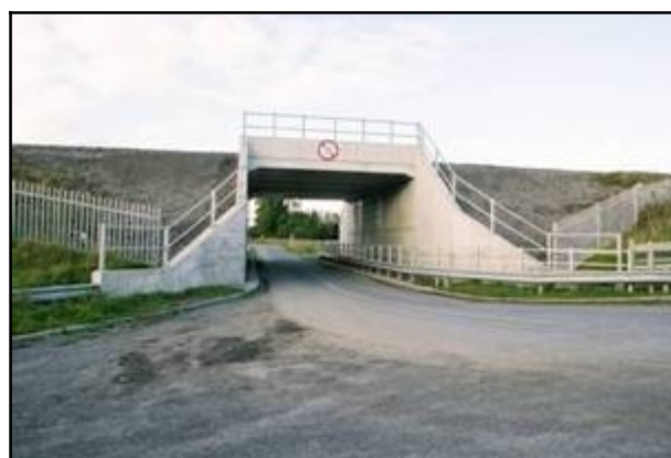
Fig 3.38a (left): Accommodation bridge at Clonyquin Td; note pre-cast concrete units on abutments and side walls (033-015). Fig 3.38b (right): Rail-over-road bridge west of Clara (008-062).
