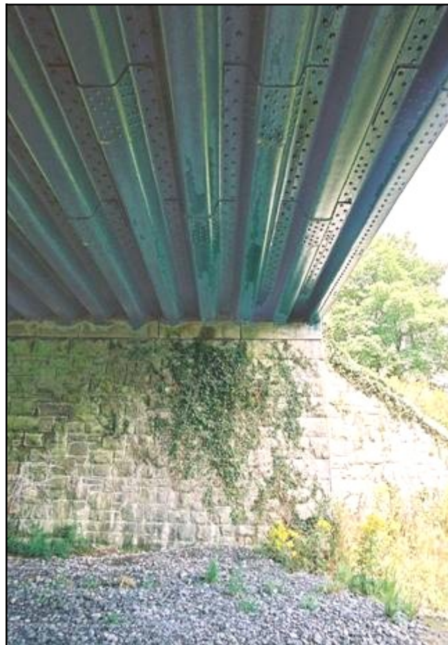
Fig 2.14a ( above left ): Late 19 th century metal girder and brick jack arch road bridge near Shannon Harbour (022-013). Note the multiple parallel metal joists, tied together with metal rods which are just visible under the jack-arch soffits.
