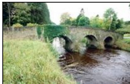
Fig 3.22 Accommodation bridge over Camcor River in grounds of Birr Castle (035-061).
