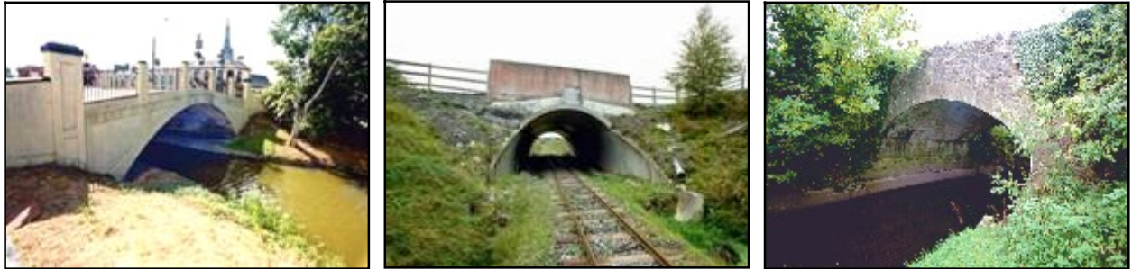
Fig 2.9a (left): Kilbeggan Bridge over the Grand Canal in Tullamore (017-016). Fig 2.9b (middle): Pre-cast concrete arch road bridge over Bord na Mona railway, Corbane Td (014-044). Fig 2.9c (right): Blackwater Bridge with concrete block voussoirs (013-005).
