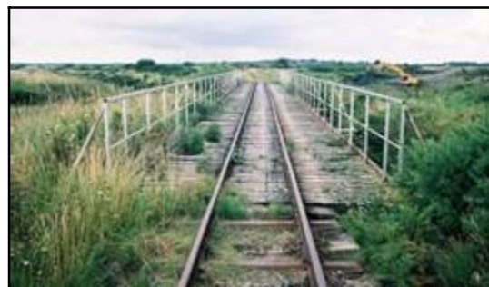
Fig 5.11 Defunct bridge carrying peat railway over Yellow River at Derrygreenagh (003-005).
