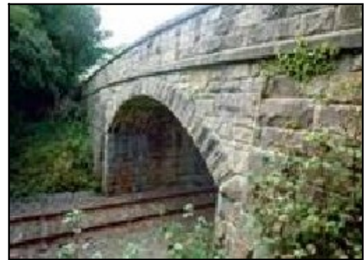
Fig 3.20 GSWR road bridge, Clyduff Td (045-010).
