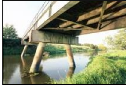
Fig 2.12a (left): Metal beam road bridge over Shannon Navigation, Clonahenoge Td (029-019).
