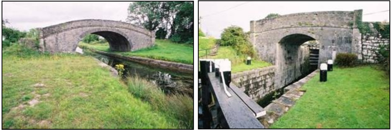
Fig 3.5a (left): Rathmore Bridge, a typical free-standing Grand Canal bridge (011-009). Fig 3.5b (right): Road bridge across the lower chamber of 33 rd lock, Belmont (014-032).
