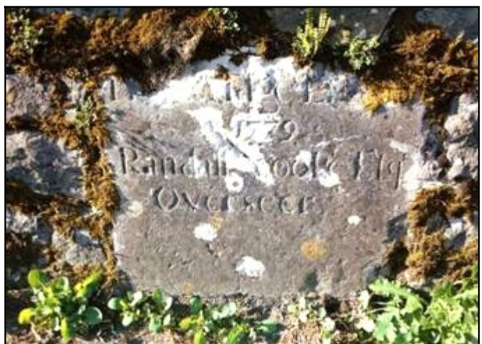
Fig 3.1 Gorteen Bridge (025-006): This bridge [laid?]/ 1779/ Randall Poole Esq/ Overseer".
