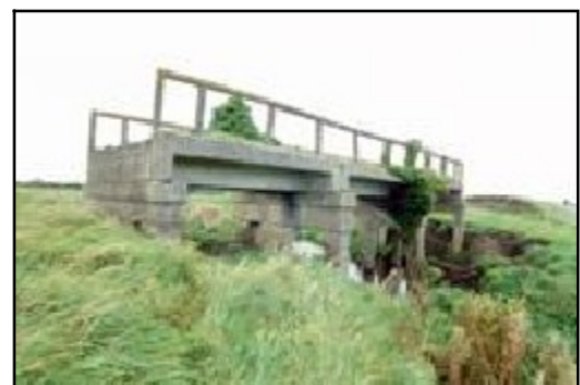
Fig 3.21 Concrete railway bridge at Clonony Beg (022-014).
