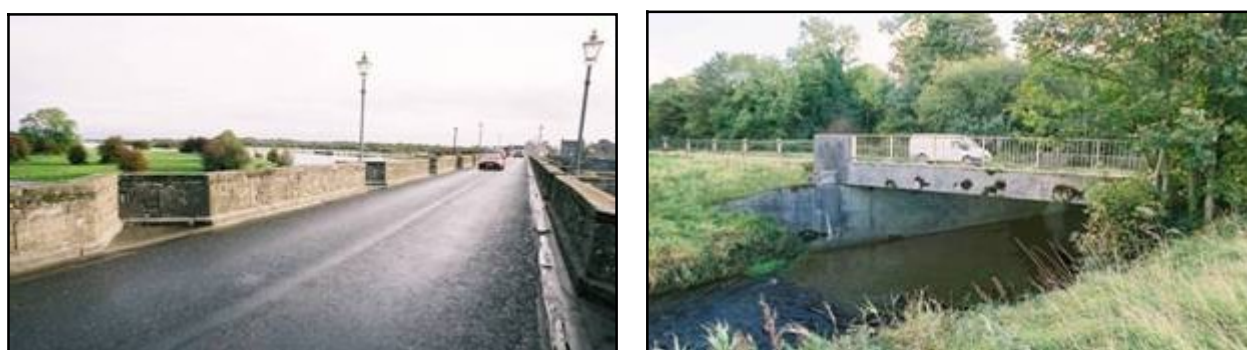
Fig 5.4a (left): Single file traffic on Shannon Bridge (013-001). Note also the pedestrian refuges along one side. Fig 5.4b (right): The new Mucklagh Bridge (016-053) on a realigned section of the Tullamore-Birr road just upstream from the old bridge (016-029).
