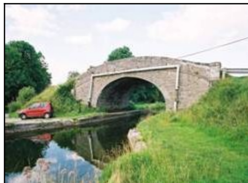
Fig 5.10 Water pipe affixed to Rhode Bridge on the Grand Canal (011-013).
