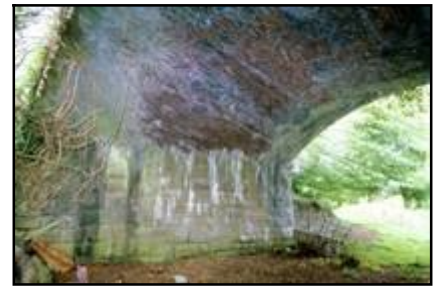
Fig 3.19 Skew brick road/rail bridge at Sharavogue (038-002).
