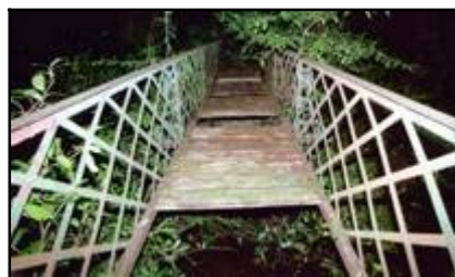
Fig 3.23 Footbridge over Camcor in grounds of Kinnitty Castle (036-026).
