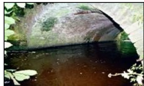
Fig 4.1a ( far left ): Architectural finesse on bridge at Kinnafad Td (004-004). Fig 4.1b ( middle ): 1649 plaque in later bridge at Birr Demesne (035-061). Fig 4.1c ( above ): Soffit breaks illustrate the progressive widening of this road bridge at Birr (035-061).
