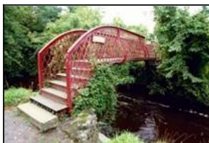
Fig 3.29a (left): Footbridge over River Brosna at Clara (008-061).
