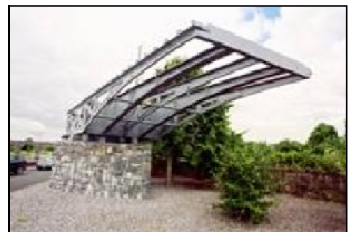
Fig 3.13 Repositioned swing bridge on Shannonbridge (013-001).
