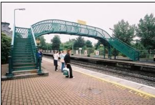
Fig 2.13a (top left): Lattice girder bridge, Glasderry More Td (042-003). Fig 2.13b (top right): Metal Bridge, Tullamore (017-002). Fig 2.13c (bottom left): Lattice girder footbridge, Tullamore Station (017-004). Fig 2.13d (bottom right): Warren truss footbridge of 1934 over Grand Canal, Tullamore (017-093).
