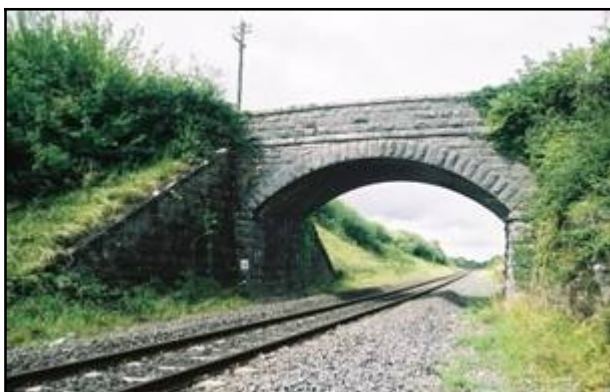
Fig 3.18a ( top left ): Skew semi-elliptical GSWR road bridge at Clonygowan (033-002). Fig 3.18b ( below left ): Orthogonal GSWR accommodation bridge at Erry (008-023). Fig 3.18c ( right ): Detailing on bridge at Erry.
