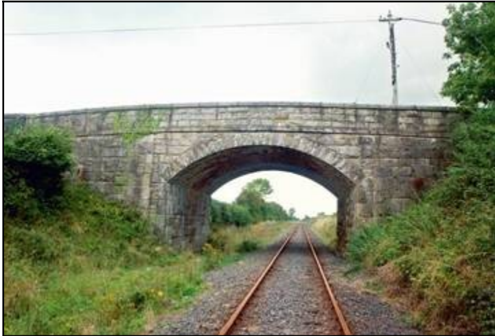
Fig 2.4a Arch bridges: masonry arch road bridge over railway, Clonlisk Td (045-003).
