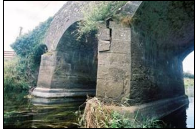
Fig 5.9a (left): Ballyboughlin Bridge (008-003) is almost totally obscured by ivy, making any structural or architectural appraisal virtually impossible. Fig 5.9b (right): Dislodged masonry at Lehinch Bridge (008-011).
