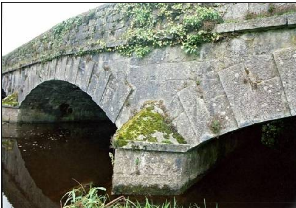
Fig 3.3 Dressed stonework on Oxmantown Bridge, Birr (035-011).
