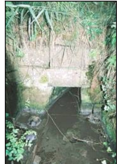
Fig 2.11 Stone drainage culvert under Kilbeggan Canal, Ballyteige Little Td (017-030)
