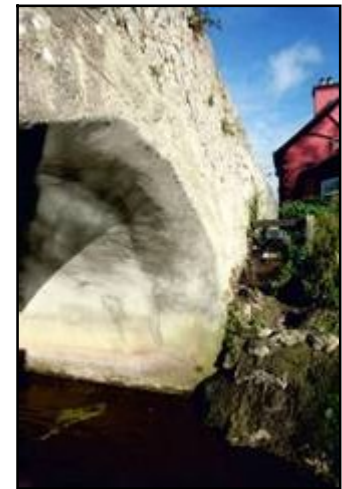
Fig 5.5 Guniting arch soffit, Riverstown Bridge (035-028).
