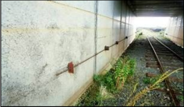
Fig 2.18a ( top left ): Kilcolgan Bridge, a beam and slab structure of c.1951 over Brosna (015-006). Fig 2.18b ( top right ): Pre-cast beam and slab bridge of 2002 over Dublin-Galway railway, Cloncoher Td (025-016). Figs 2.19c and 19d ( bottom ): This pre-cast concrete box-section bridge of 1999 carries the Daingean-Tullamore road over a Bord na Mona railway (018-041). The individual units are tied together with metal rods.
