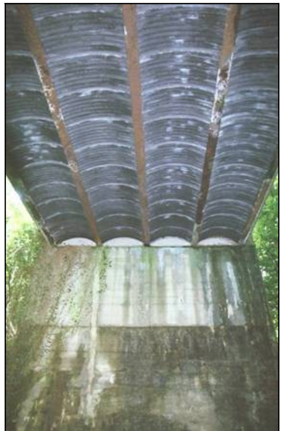
Fig 2.14a ( above left ): Late 19 th century metal girder and brick jack arch road bridge near Shannon Harbour (022-013). Note the multiple parallel metal joists, tied together with metal rods which are just visible under the jack-arch soffits.
