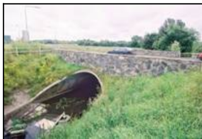
Fig 3.28a (left): The c.1850 bridge built by the Board of Public Works (012-004).
