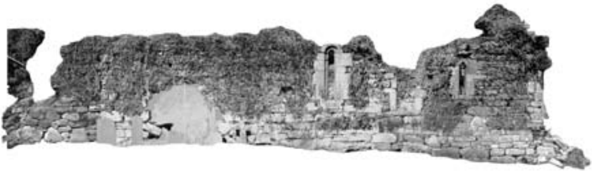
South wall external
