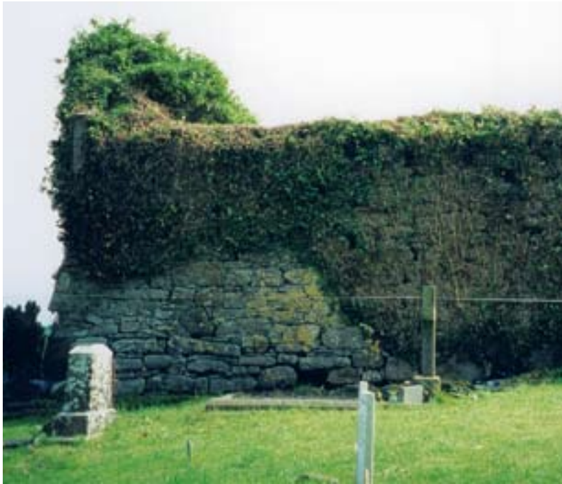
Plate 12: The North Wall [Project Team May 2001 – January 2002]
