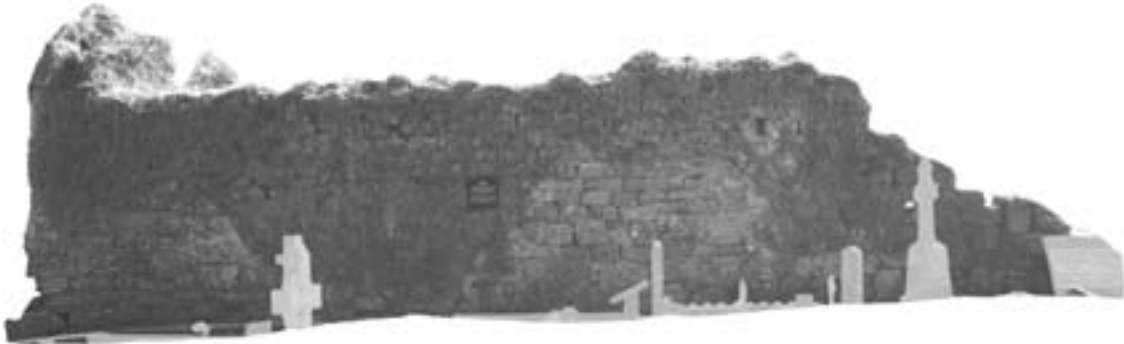
North wall external
