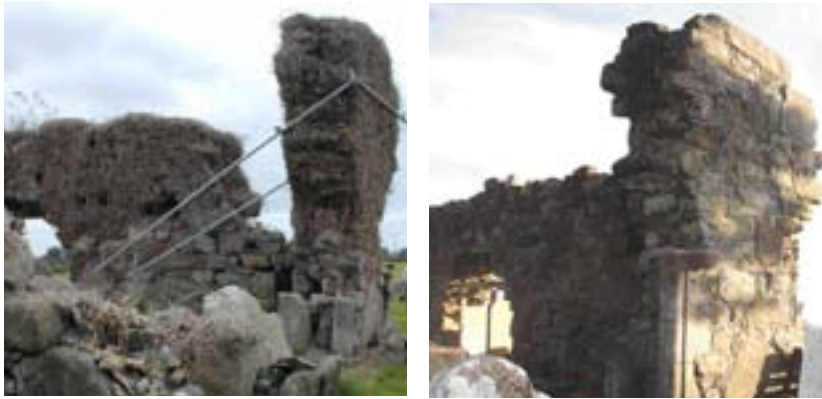
West gable before and after repair
