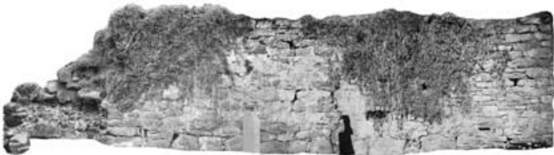
North wall internal
