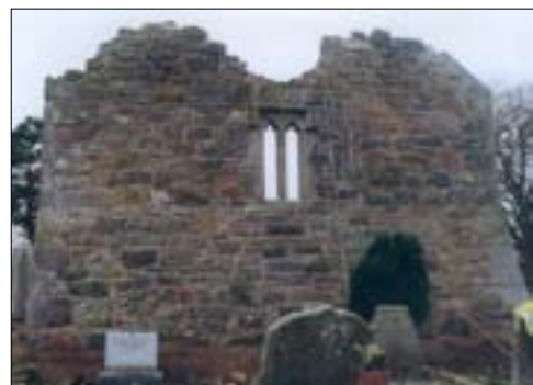
East gable following repairs
