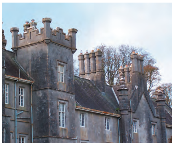
Roof detail, from north-east
