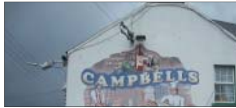
Townsend Street: Cabling causing visual clutter
