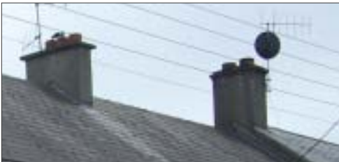
Townsend Street: Multiple antennas visible from the street
