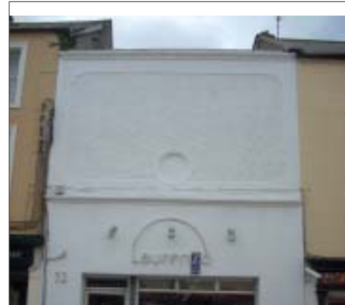
Main Street: Taller shop front breaks building line
