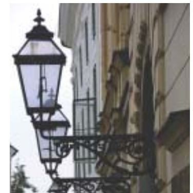
Example of street lighting fixed to building to reduce street clutter
