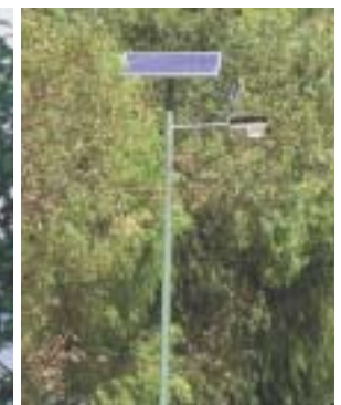
Solar powered street light to be used in newer developments
