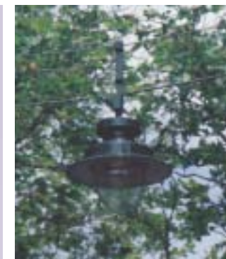
Cantenary lighting with similar lantern style works in narrow streets and reduces clutter
