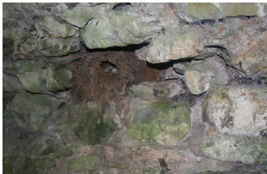
Fig 1.1 Dipper nest in bridge cavity Weir Bridge, River Little Brosna
