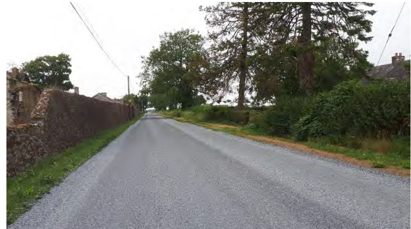
1km Surface Dressing scheme at Moystown
