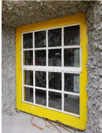
Steel window repair, Derrybeg
