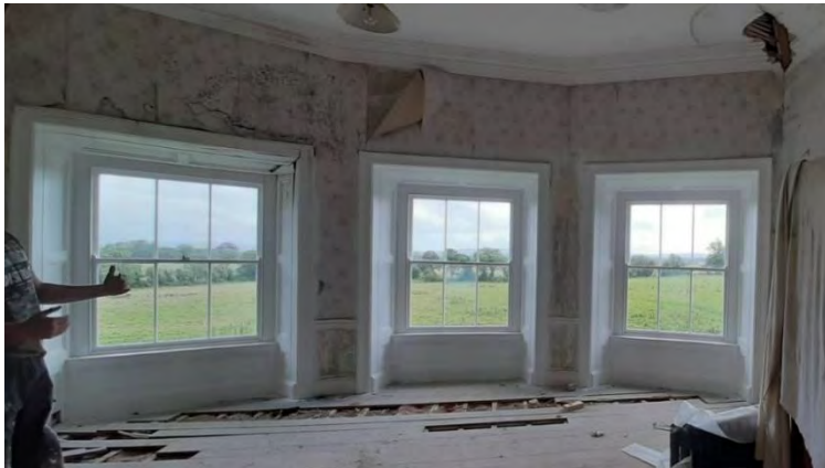
Detail of some of the metal windows set in a timber frame
