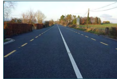
Photo: N80 Tullamore to Derryclure Pavement Renewal
