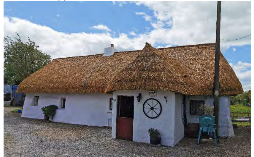
Thatch repairs to second Derrybeg site
