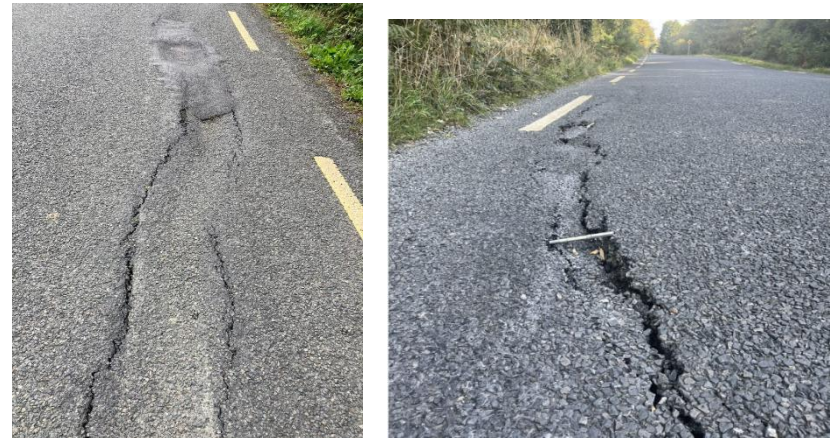
Examples of Peat Road Failures that occurred in Q3 2022
