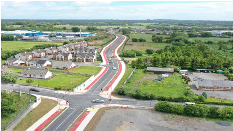
Aerial View of the Edenderry Inner Relief Road
