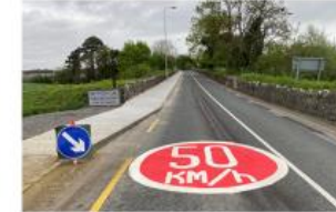
Photo: Portarlington - New footway to Cemetery
