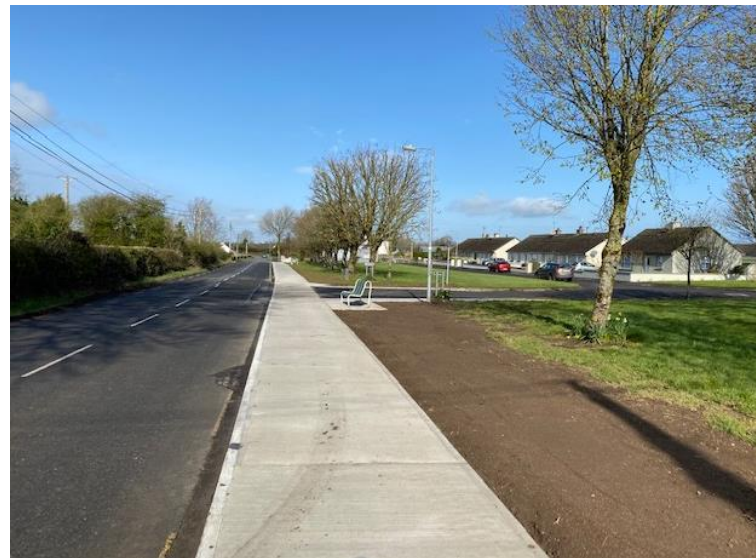
New footpaths at Ballincur in Kinnitty were constructed using Active Travel Funding in 2021
