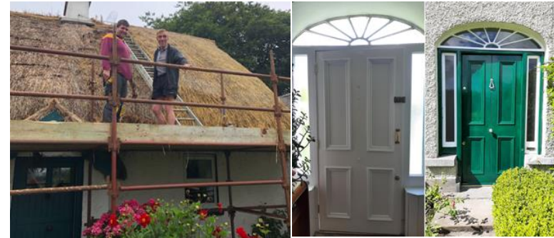
Thatch Repairs Cappincur Door Repairs Birr
