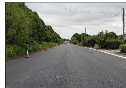
Photo: N52 Ballinacard East & West Pavement Scheme
