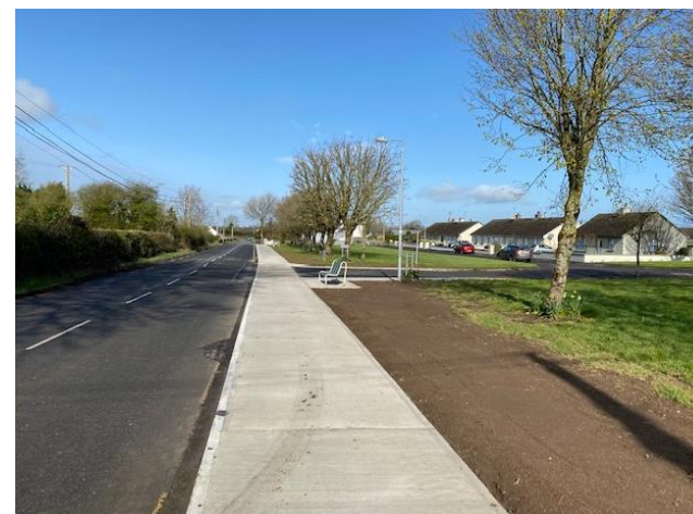
New footpaths at Ballincur in Kinnitty were constructed using Active Travel Funding in 2021
