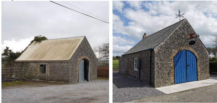
Killyon Forge, Before and after works
