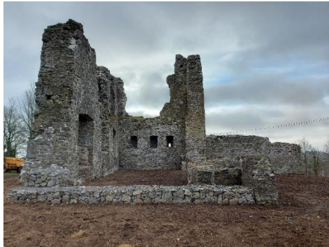
Blundell Castle, Edenderry, December 2021 post conservation works
