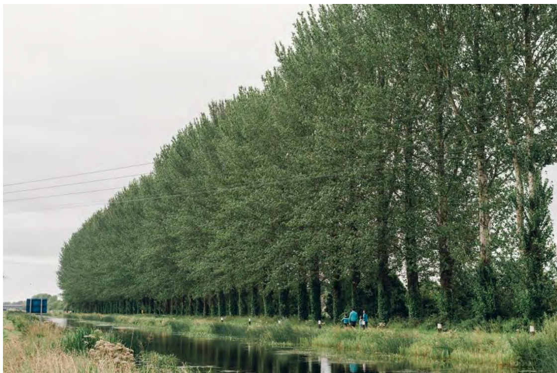
Figure 9.1. Grand Canal Greenway, Co Offaly
