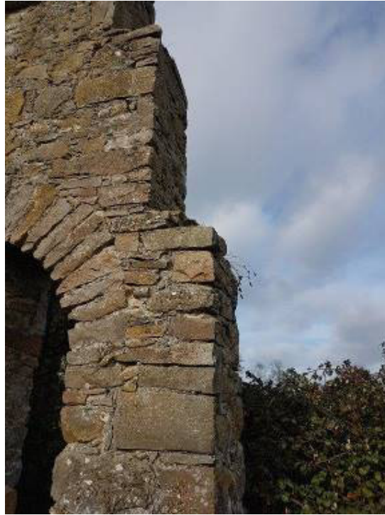
15. Evidence of previous sloping stonework is found in one location
