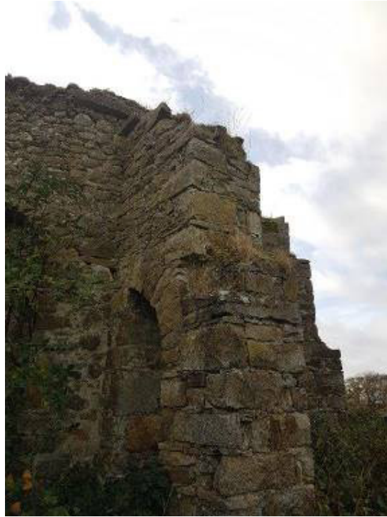
3.1 The following photos are taken of the exterior clockwise
