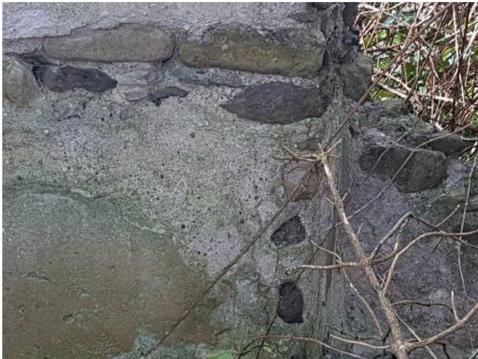
11. Close up of stonework.
