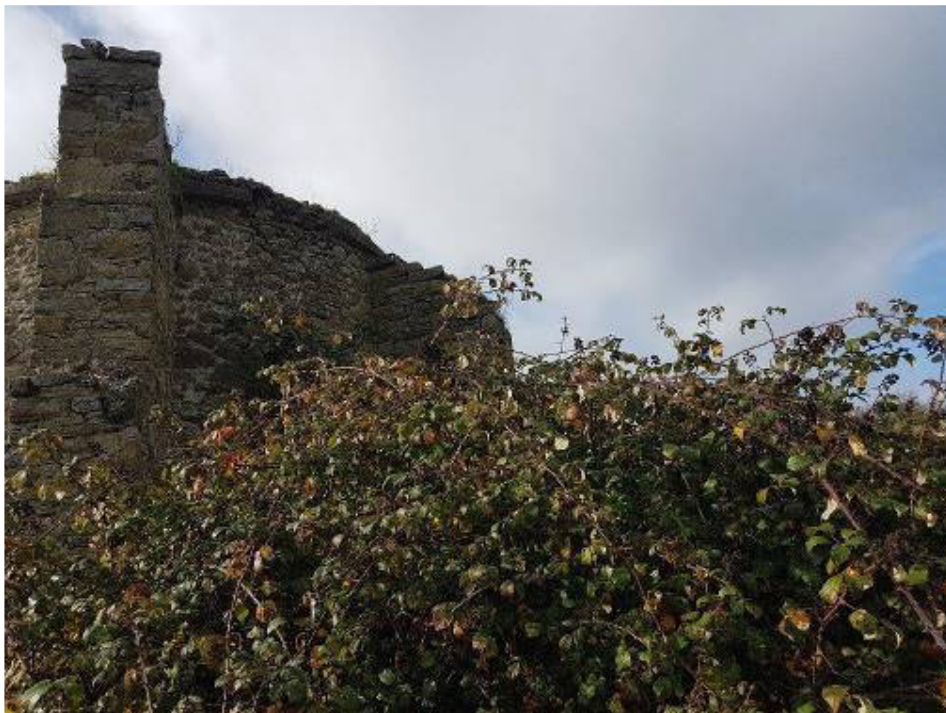
2. Exterior stonework in reasonable condition. Area around to be cleared
