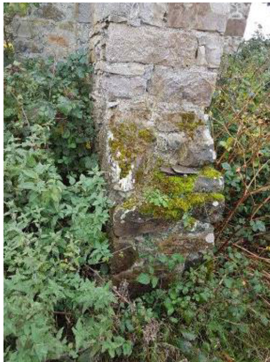
15.1 Sloping masonry to bottom of buttress.
