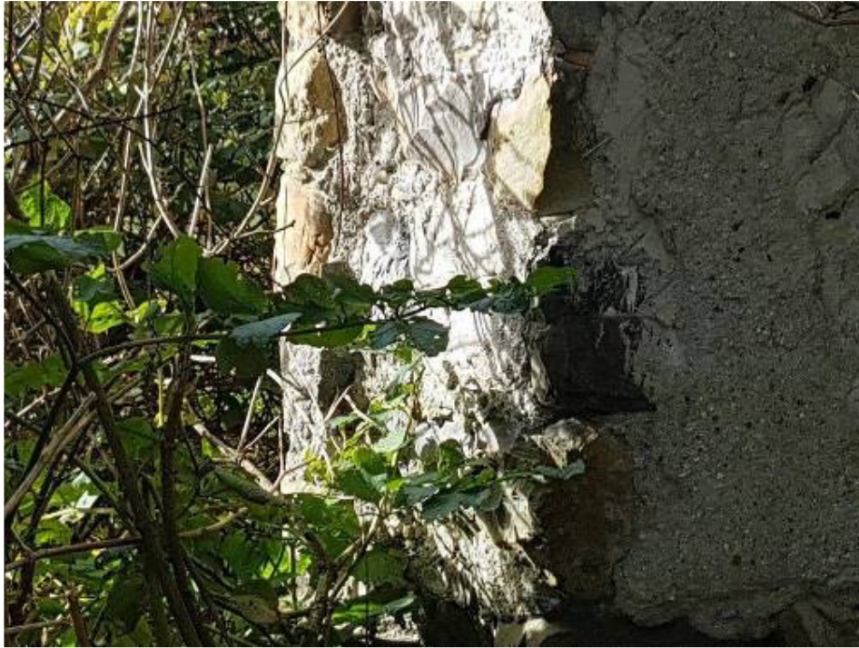
16. Typical window reveal implies working sash windows in the past.
