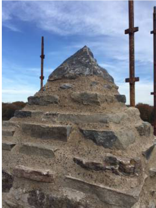
Suggested termination of top of pinnacles
