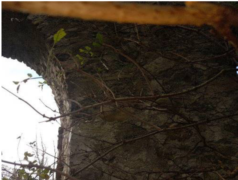
5. Arch voussoirs in reasonable condition.
