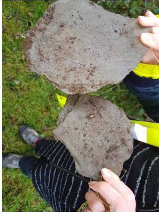
4. Evidence that roof was slated.
