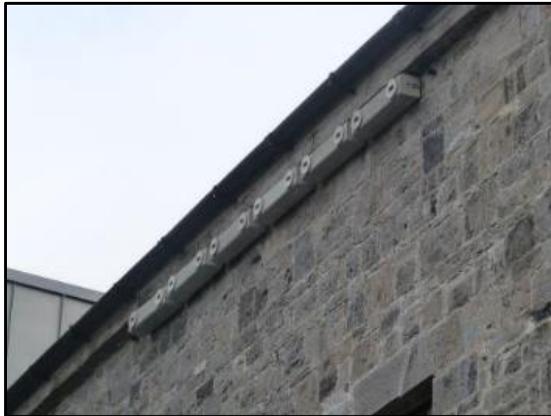
Figure 31. A row of Swift nest boxes installed at Mullingar Courthouse. Photo: Richella Duggan.
