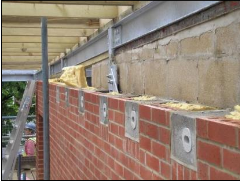
Figure 33. Swift Bricks installed during build phase in Nothing Hill, London.
