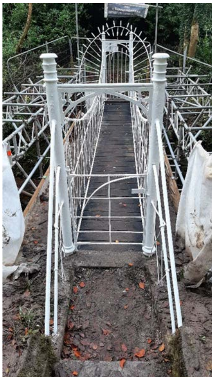
Castle side with full height gate and spear finials in place
