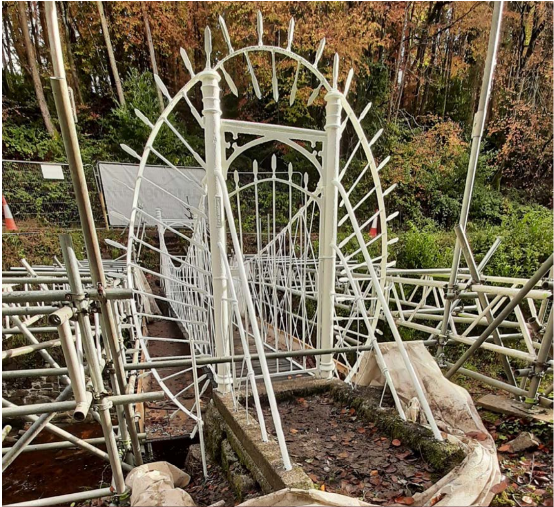
Castle side with full height gate and spear finials in place
