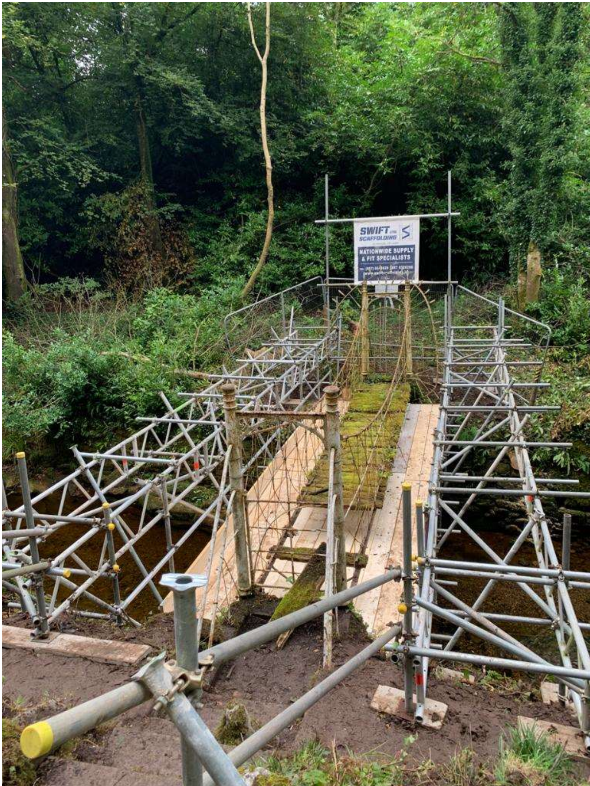
Scaffolding built around bridge with first layer of support below deck
