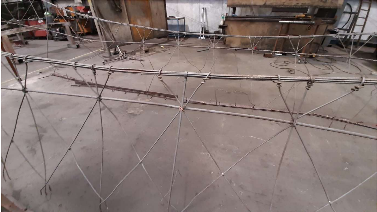
Diagonal bracing (lower) to be extended by TIG welding. All original components to be retained (CS)
