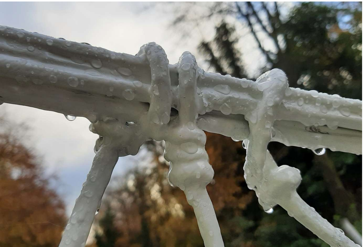
Freshly painted diagonal and horizontal connections to top chord
