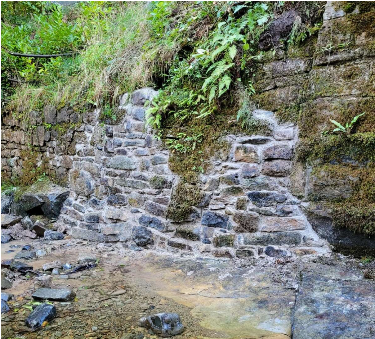
Embankment built up and secured with lime mortar
