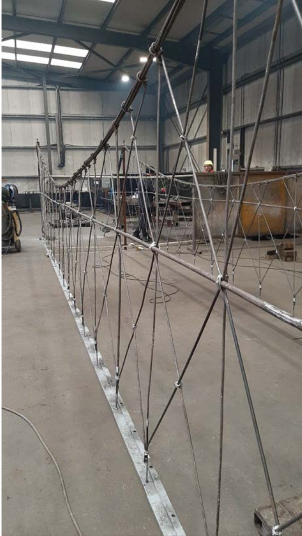
Bridge repairs underway
