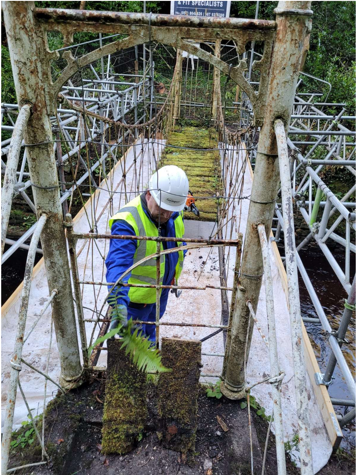
Existing pedestrian swing gate to bridge
