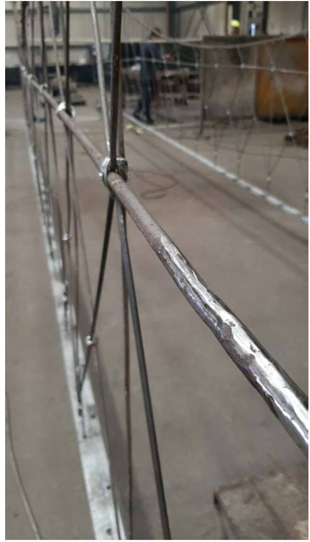
Welding new sections where required to horizontal rail
