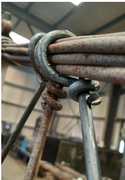
Replacement and original sections
