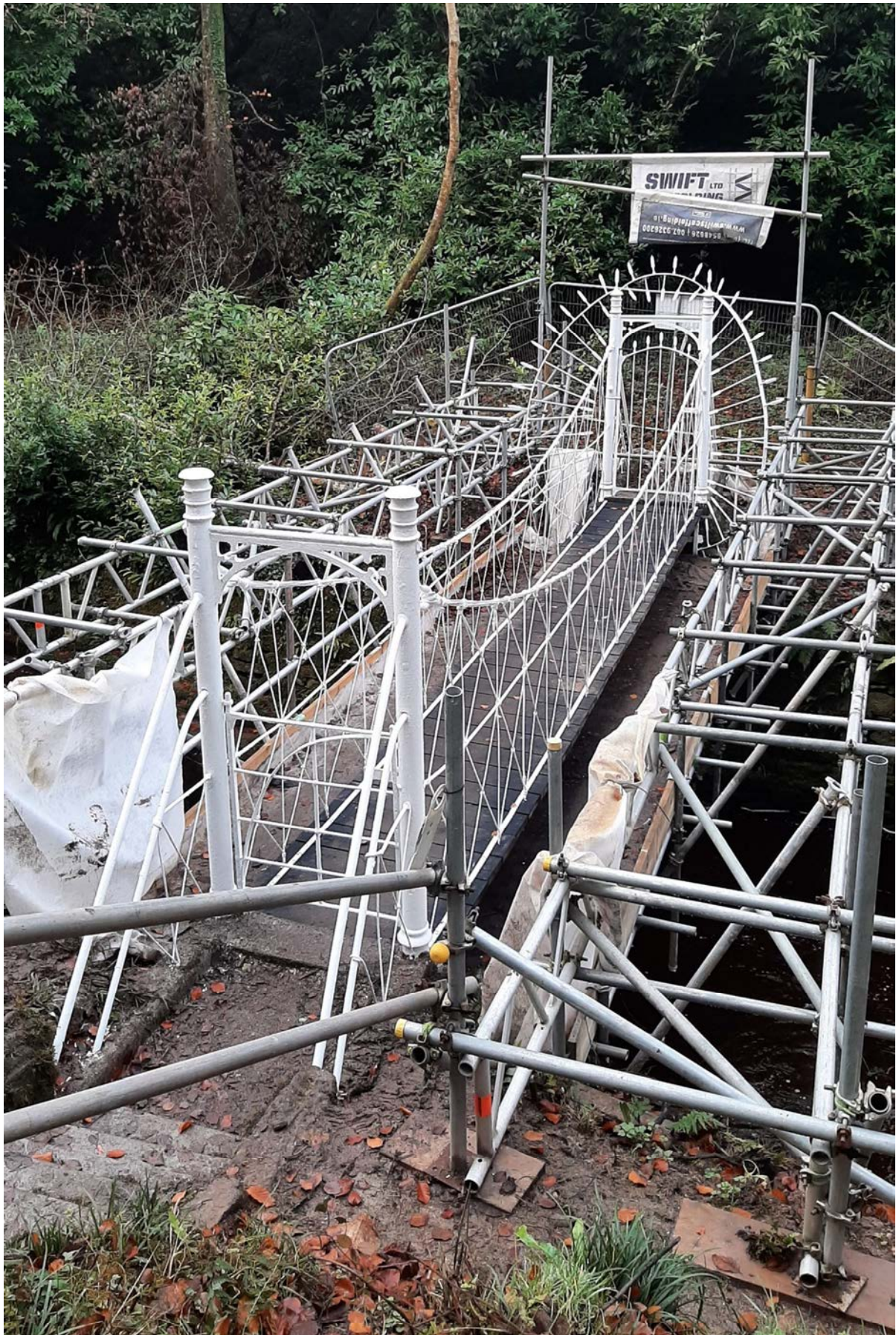
2021_1115 Suspension Bridge back on site
