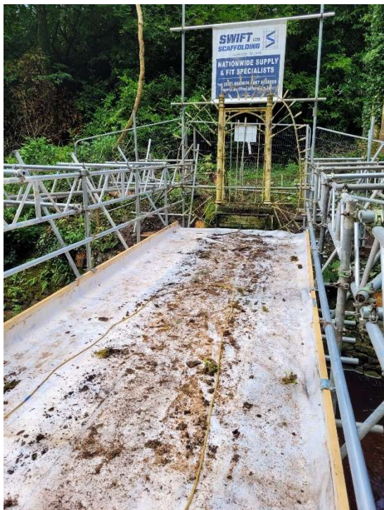
Temporary support below and around the bridge
