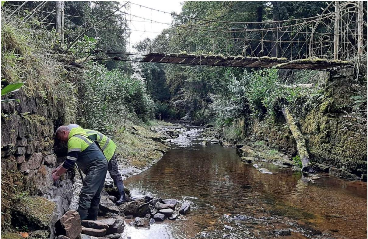
Loose stones washed down river, returned and set in lime mortar
