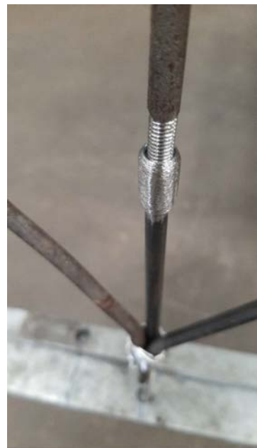
Threaded fixing to coupler
