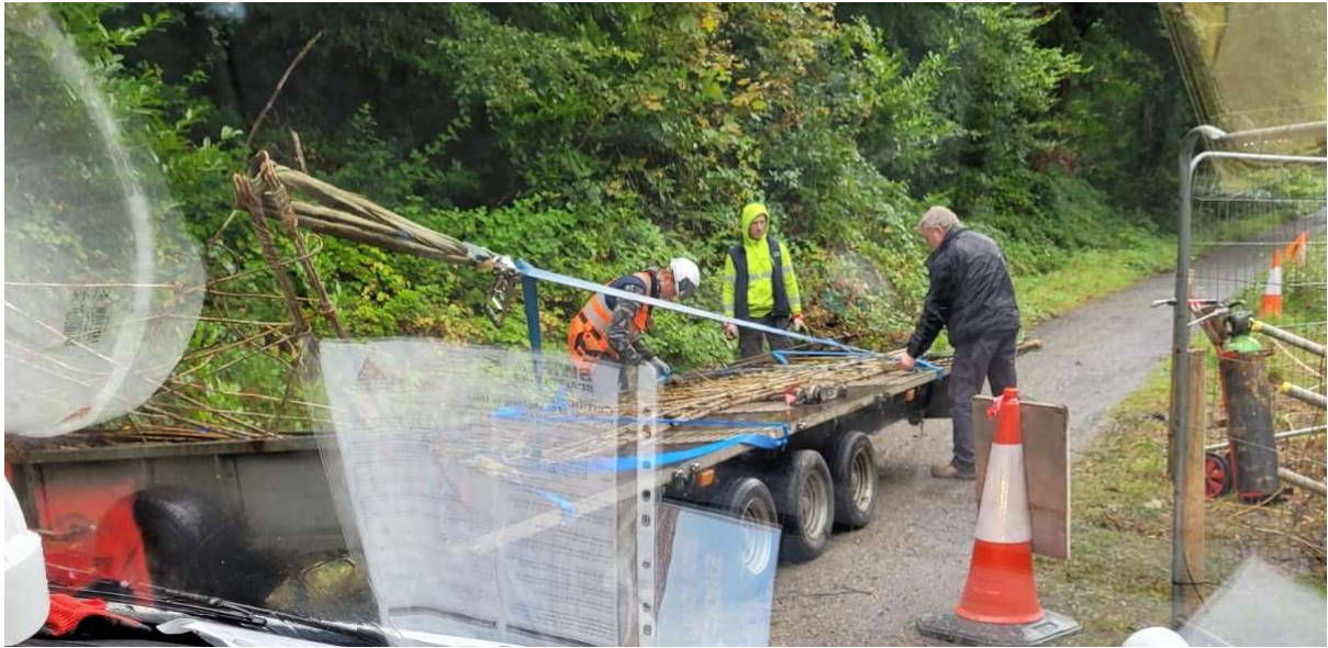
Preparations for removal
