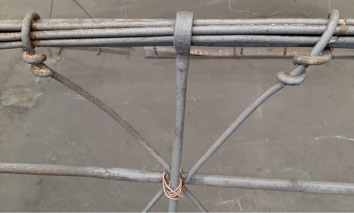
3 No 10mm uprights each side to be extended with M10 couplers (CS)
