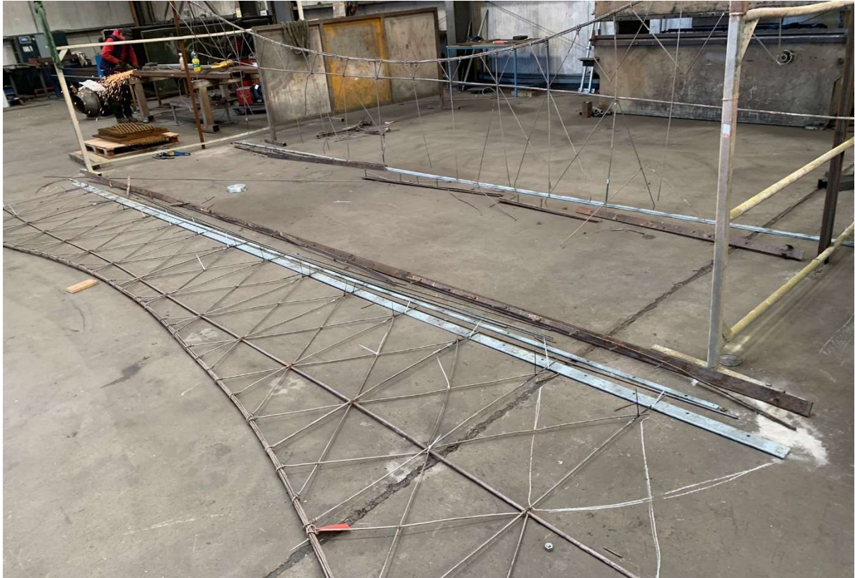
Workshop images: 2021_1022 New bottom rail prepared to take existing supports
