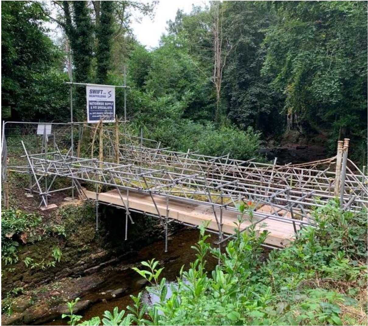
Temporary support below and around the bridge
