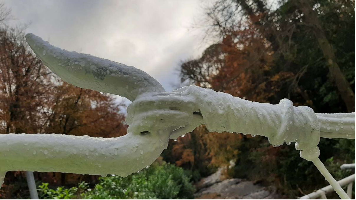
Top chord fixing detail to uprights
