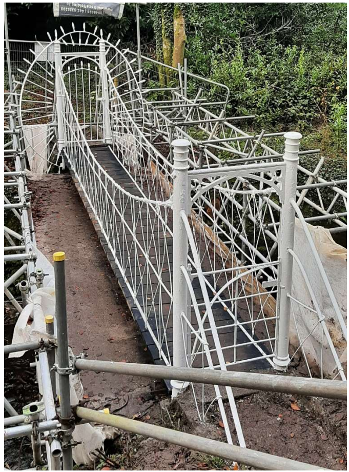
Back in place, repaired and conserved
