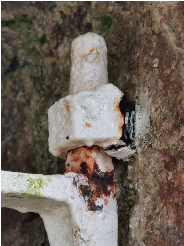
Wall fixing top and bottom. Loose bars (below)
