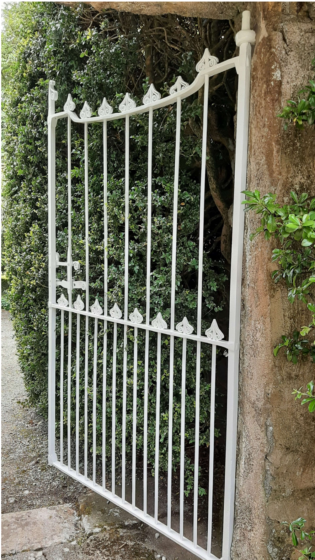
2021_0818 Site photos of completed project
