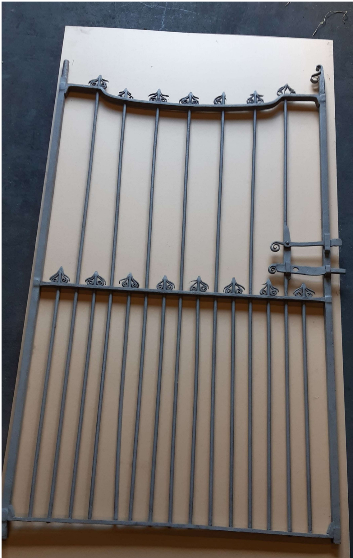
2021_0615 Blacksmith images – Gate taken off site, paint removed to prepare for repairs
