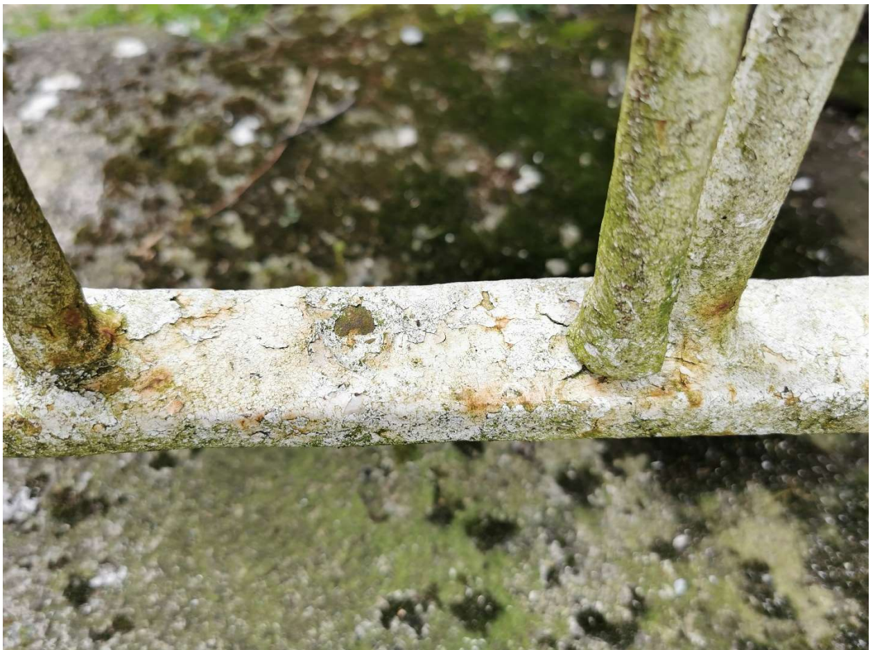
Wall fixing top and bottom. Loose bars (below)
