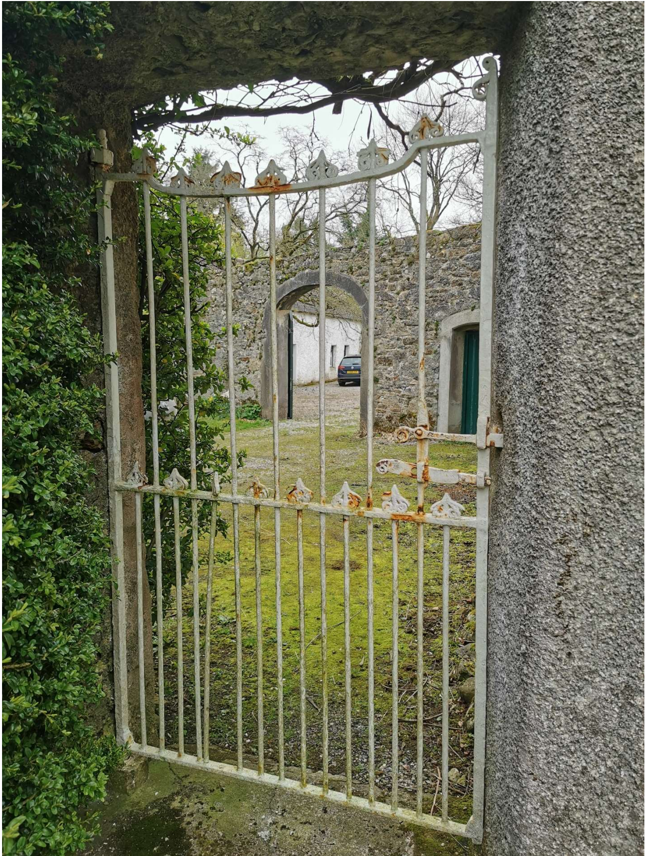
Woodfield Gate prior to works
