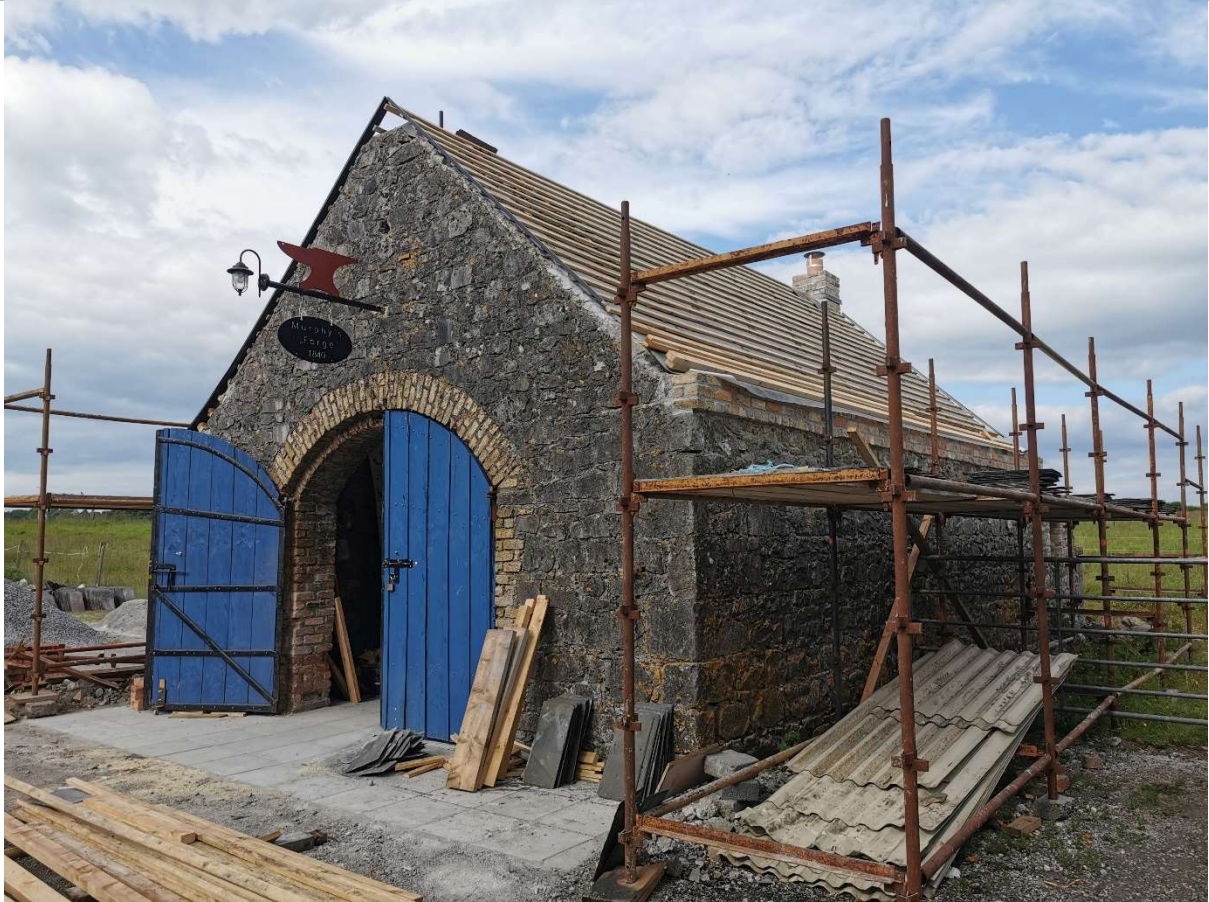
2021_0618 – Natural slate roof commences
