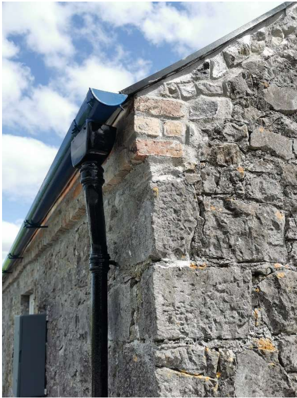
Gutters, downpipe and brick corbel detail
