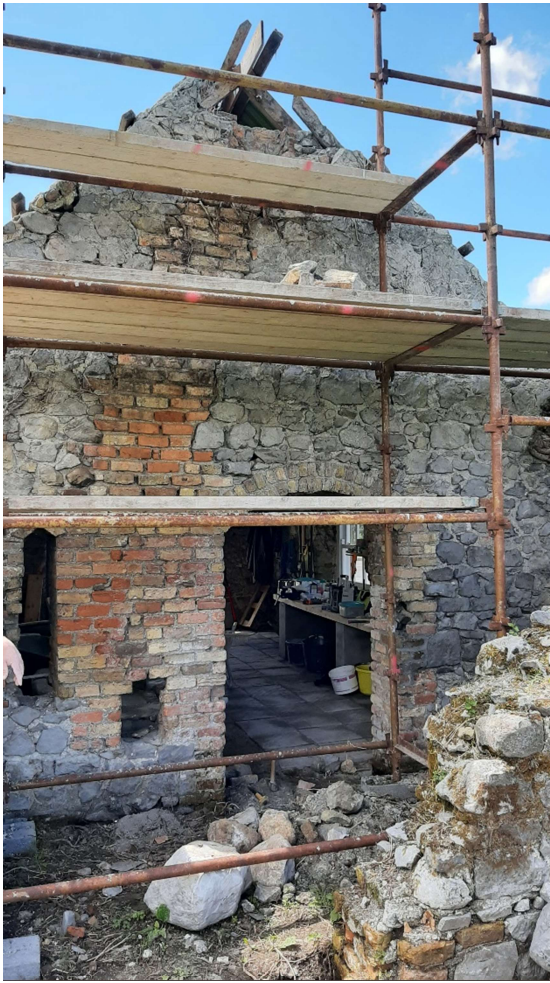
Gable repairs, brick and stone underway, retaining all openings and brick or pointed arched detailing, corrugated metal roof removed
