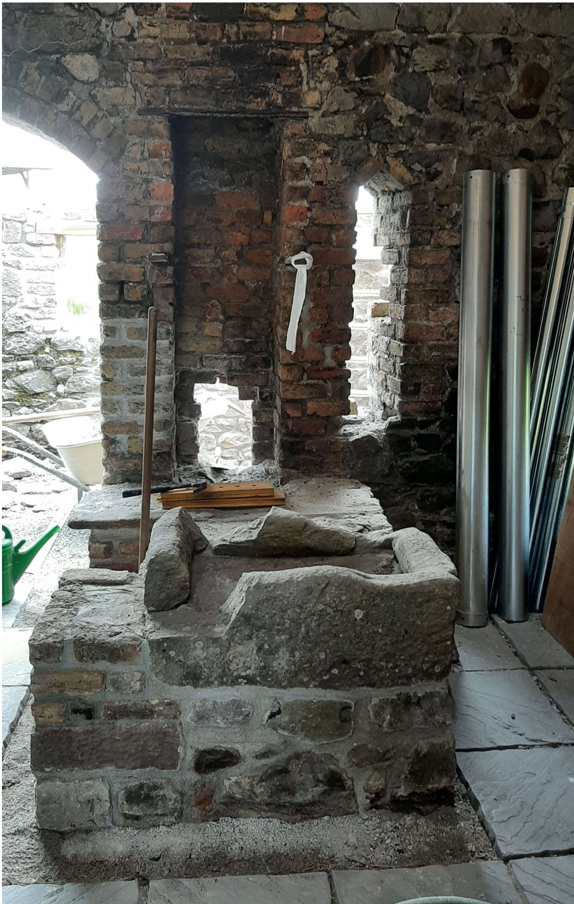
Internal repairs to blacksmith fixtures
