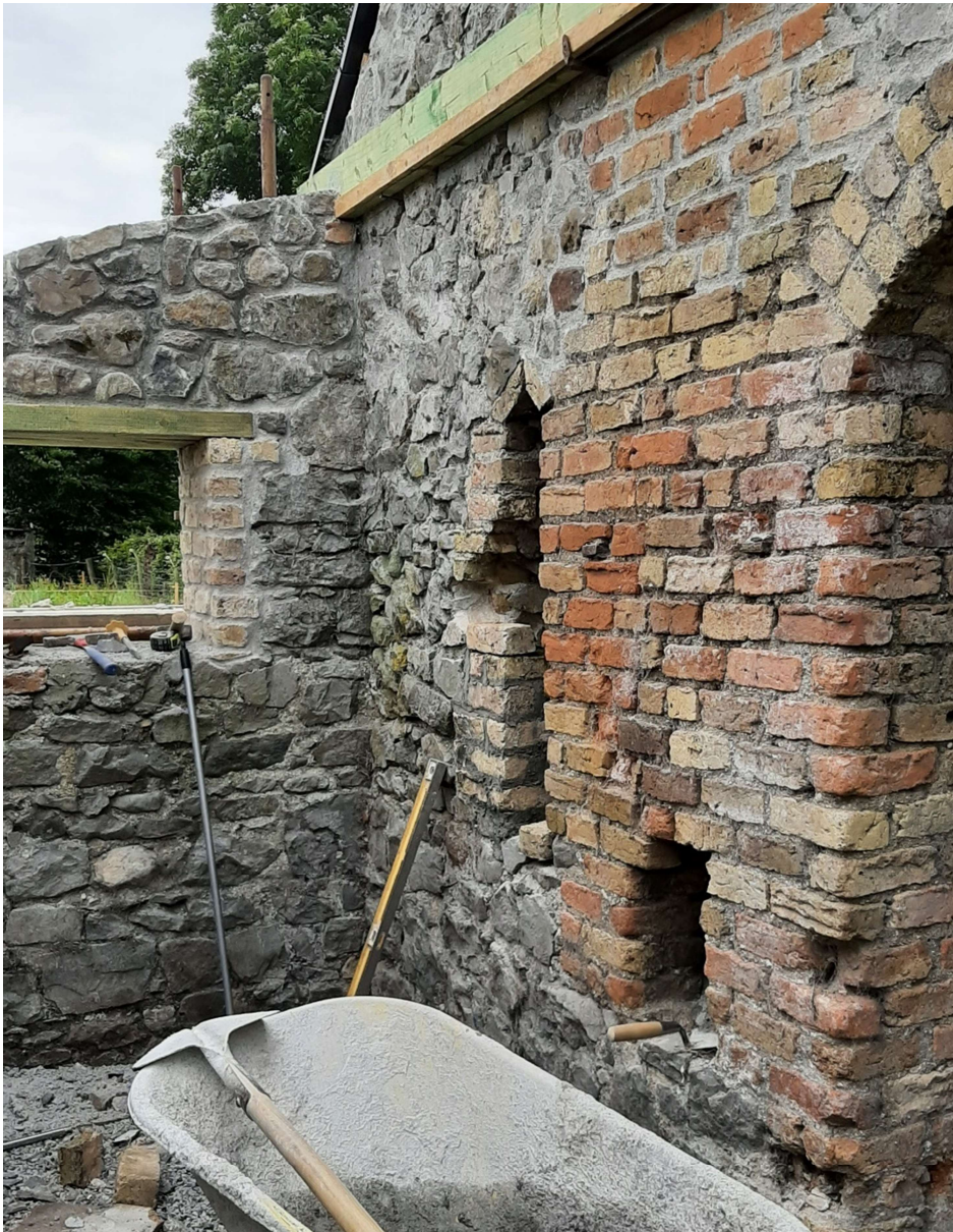
Repairs to brick arched openings, vents, windows and lean-to at rear
