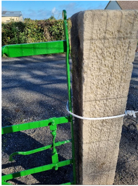
Owner photographs – workshop detail and installing repaired gate on site.
