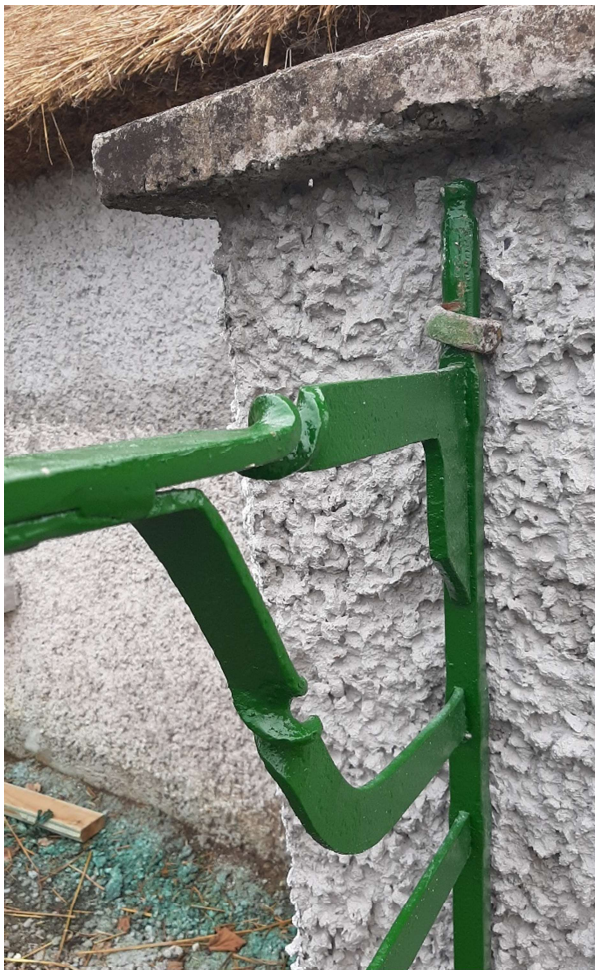
Original pier re-dashed to match house, bracket detail + Fixing detail
