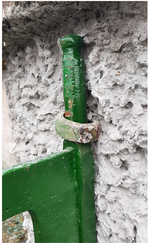
Original pier re-dashed to match house, bracket detail + Fixing detail
