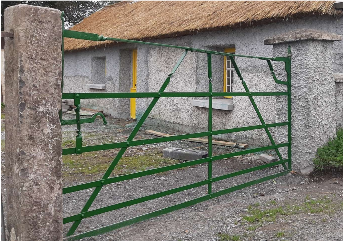
Gate repaired and installed with cut stone pillar found on site
