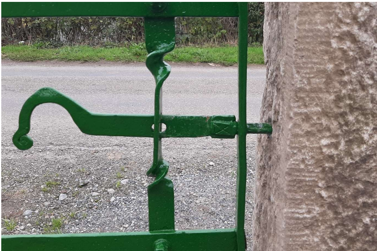
Latch detail with curved handle and scroll finial. Note blacksmith mark (X) at latch bar.
