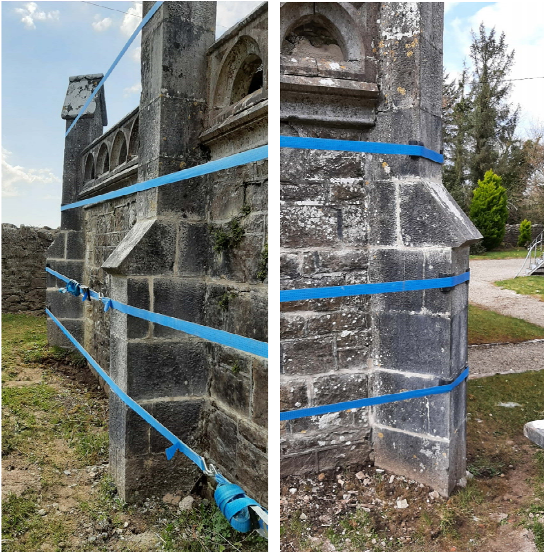
Kneeler stones returned and surrounding joints repaired with lime mortar
