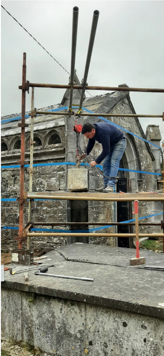
Kneeler stone carefully removed, for plate. Plate and tie-rod inserted 05 April 2022
