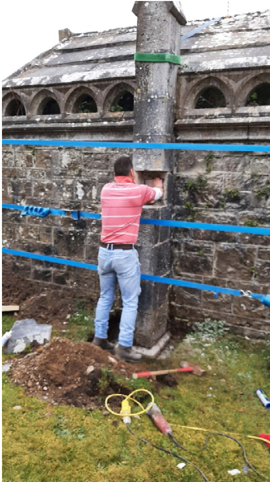
Steel rod and plate underway to buttress and new underpinning, 30 March 2022
