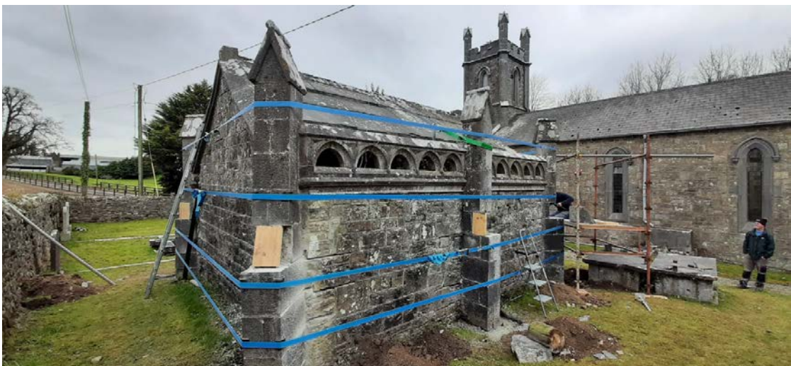
Kneeler stone carefully removed, for plate. Plate and tie-rod inserted 05 April 2022
