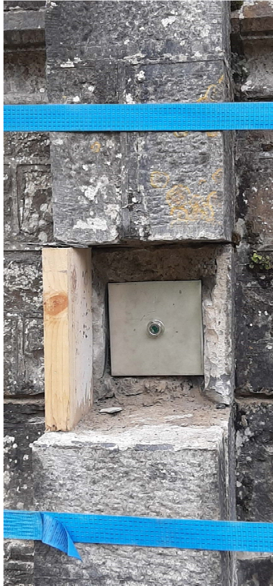
Kneeler stone carefully removed, for plate. Plate and tie-rod inserted 05 April 2022
