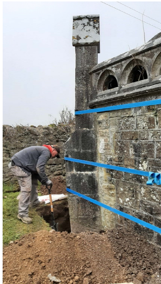
Steel rod and plate underway to buttress and new underpinning, 30 March 2022
