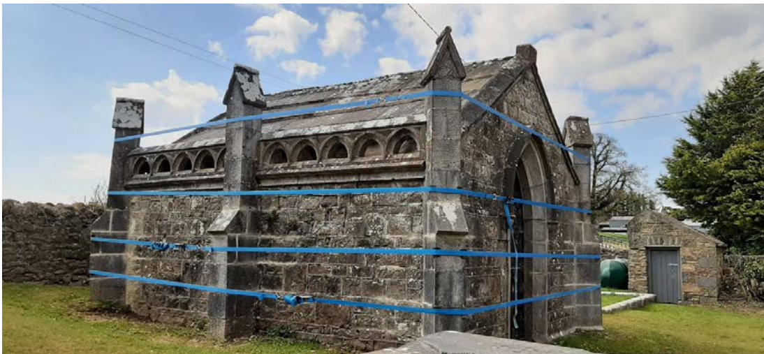
Kneeler stones returned and surrounding joints repaired with lime mortar
