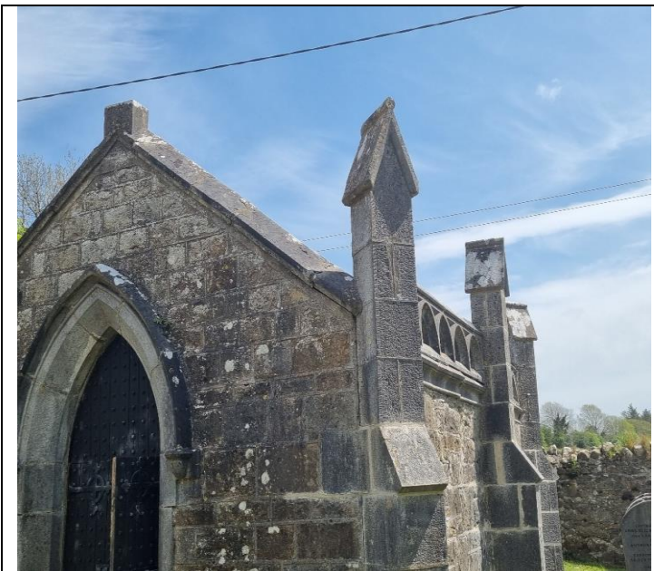
3. The decorative stonework was attached
