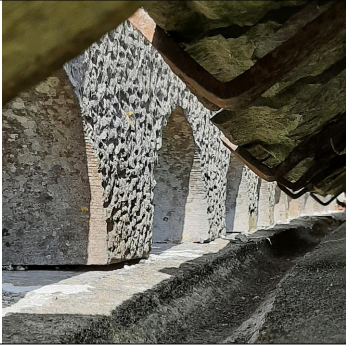
13. The valleys have been cleared and cleaned of debris, the joints pointed in an NHL 5 and the finished surfaces protected in a Remmers water repellent
