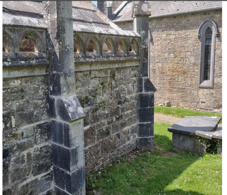
10. Repointed joints with crack tie reinforcement will be coloured to match existing
