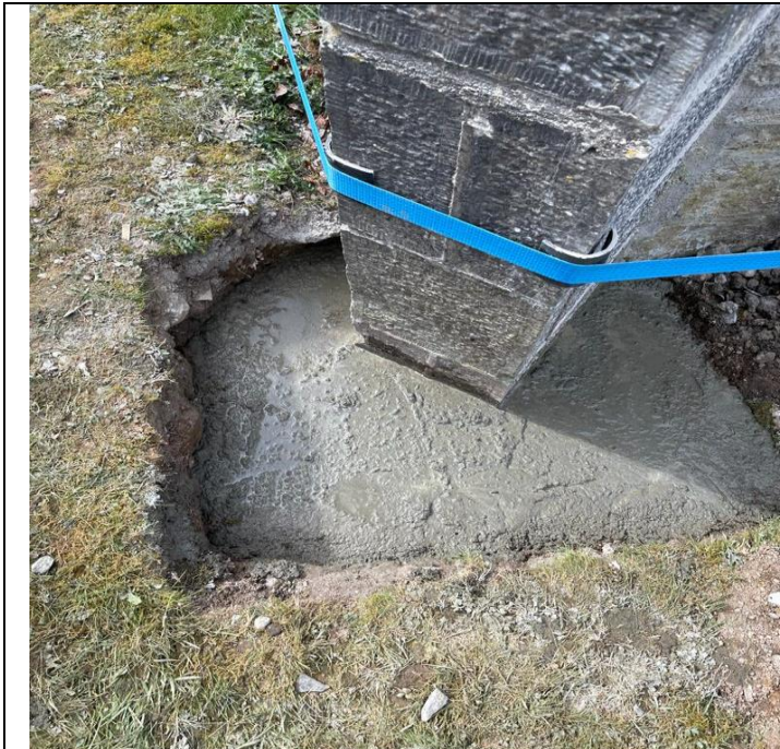
11. Underpinning works during the project stabilising the base of each buttress
