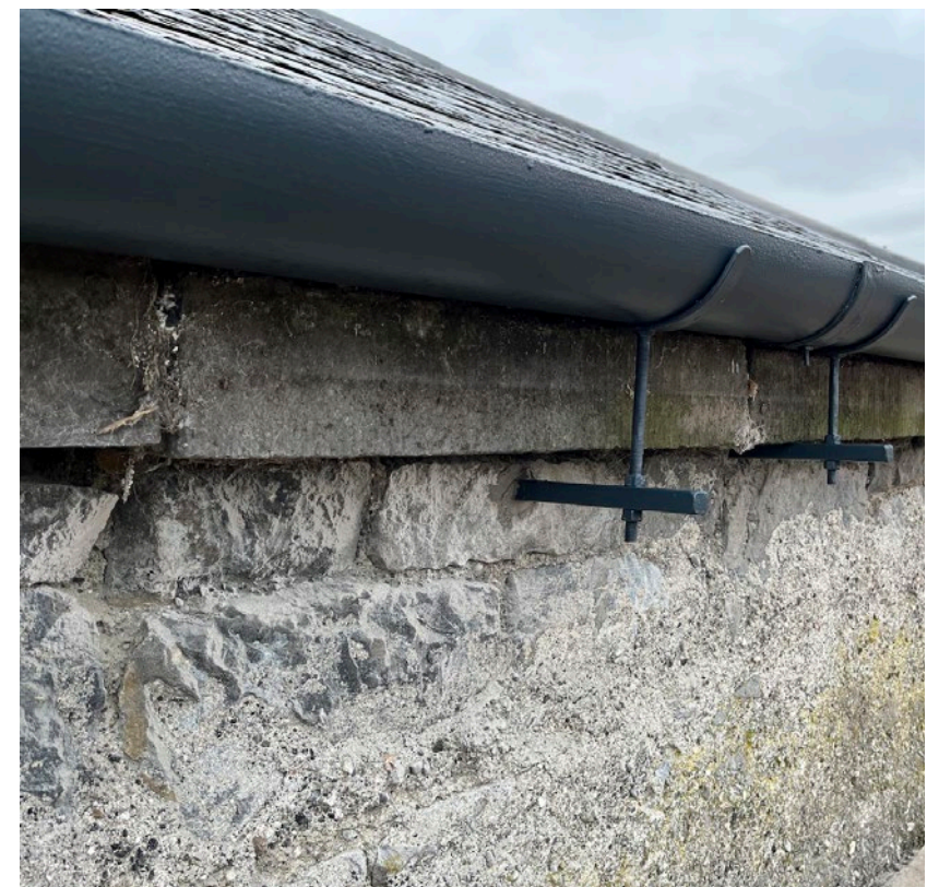
Figure 17 - Tooled eaves stone to roof
