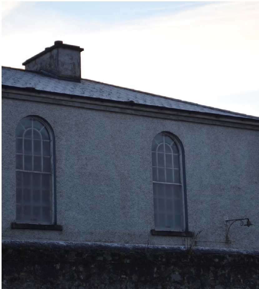
Figure 21 - North facade windows
