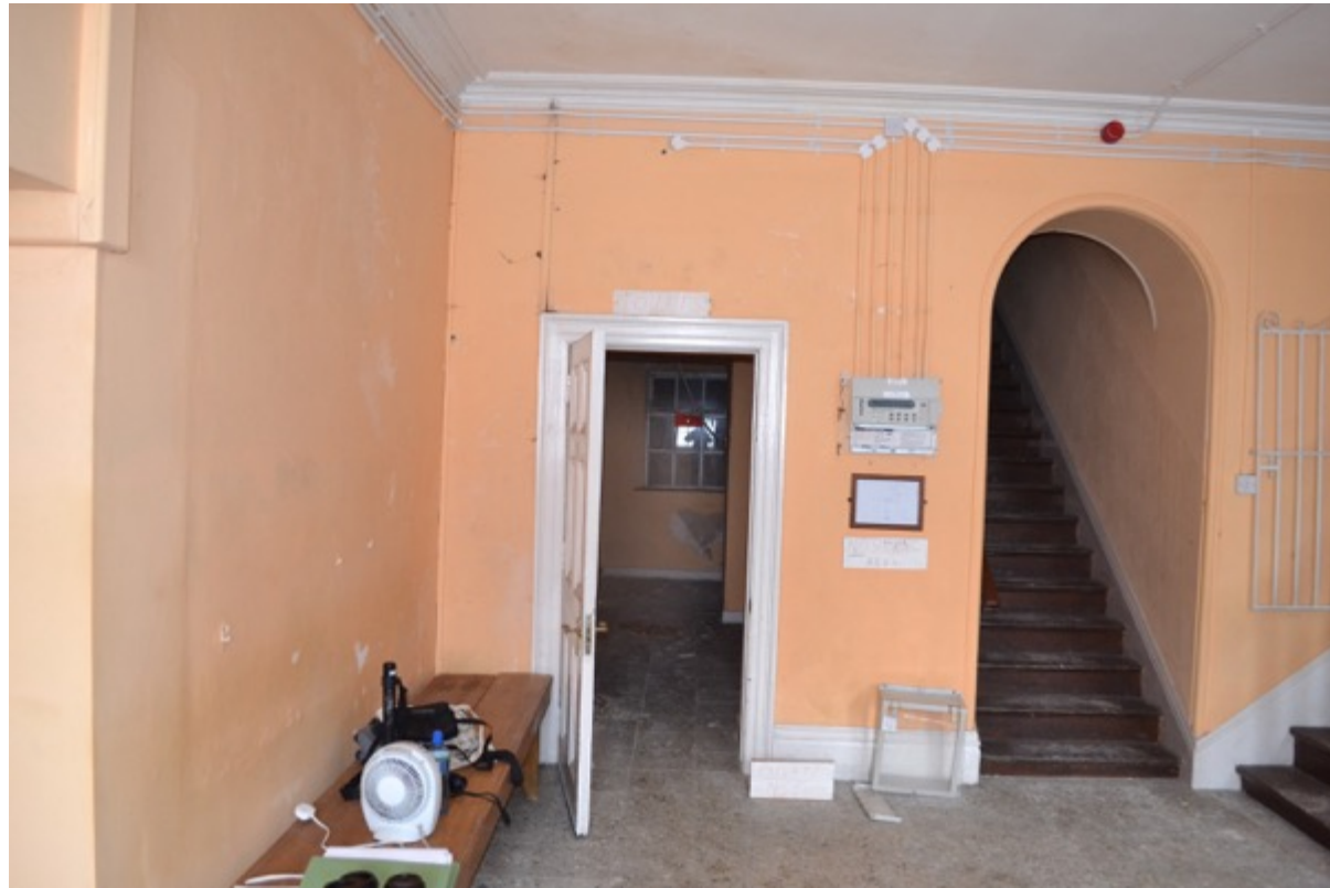
G02 – Reception – stair to rear extension on right
