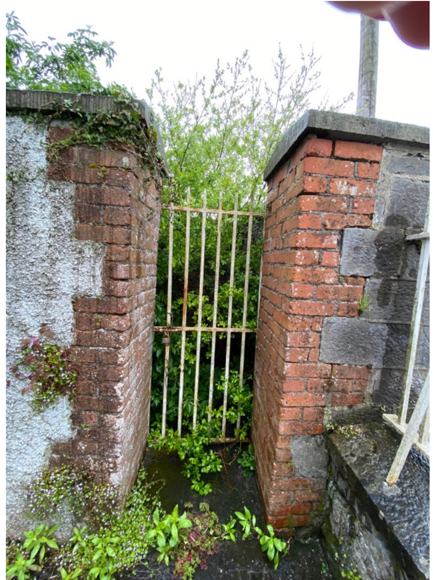
External Plant Enclosure
