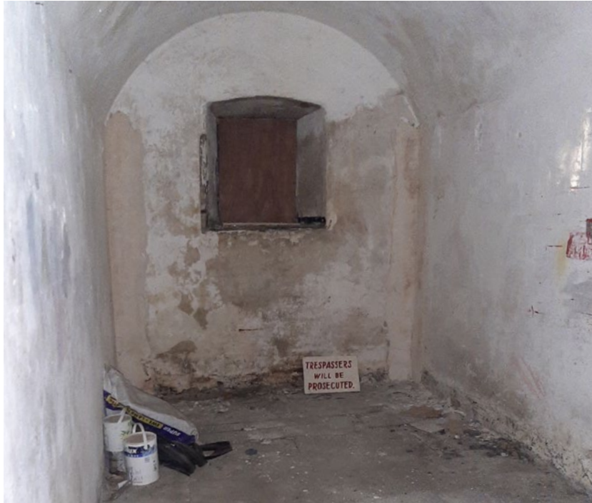
Figure 31 - Plastered vaulted cells
