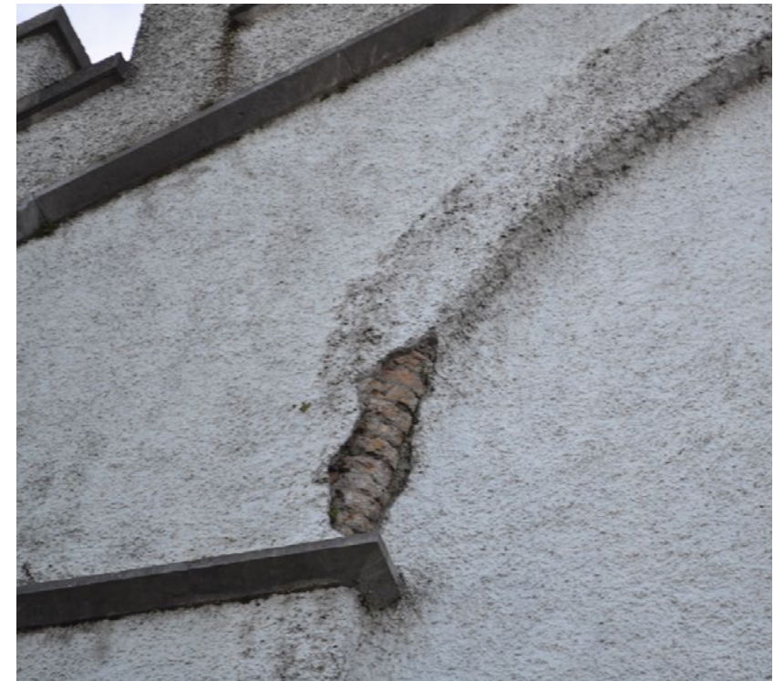
Figure 18 - Exposed brickwork beneath the cement render on the front facade
