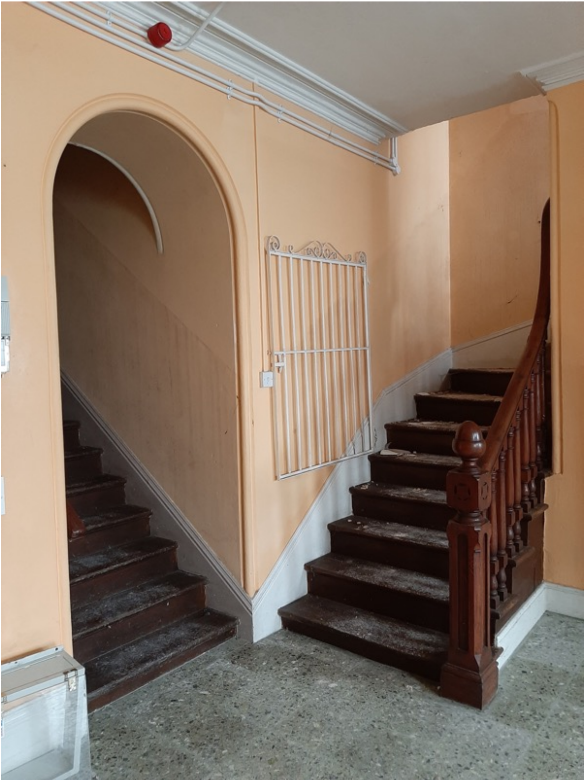
G02 – Reception – stairs to rear extension and to courtroom mezzanine
