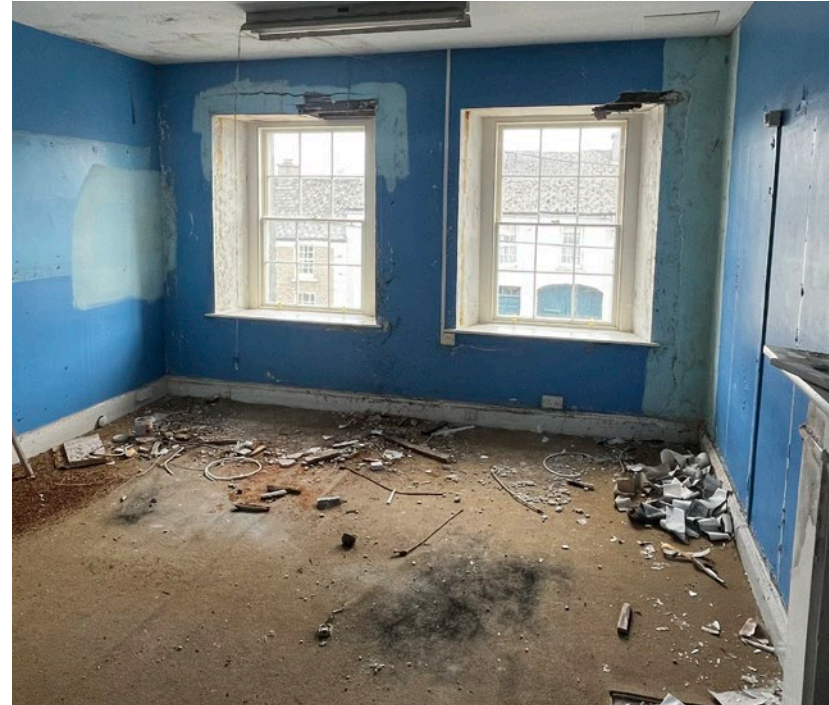
Figure 30 - Internal view of the front room at first floor level
