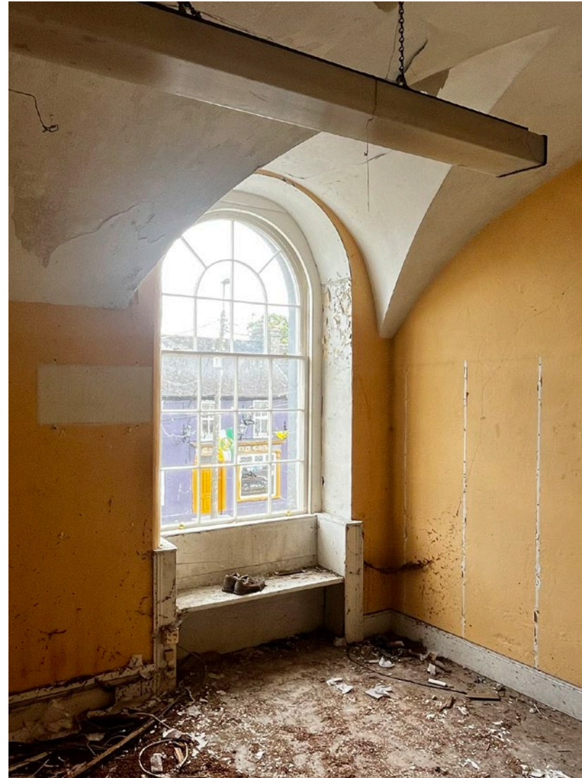
Figure 12 - Existing spoked timber sliding sash window
