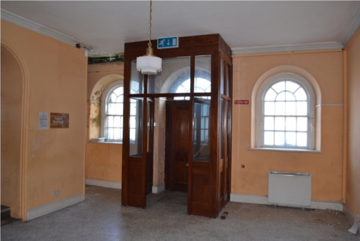
G01 – Timber frame Lobby
