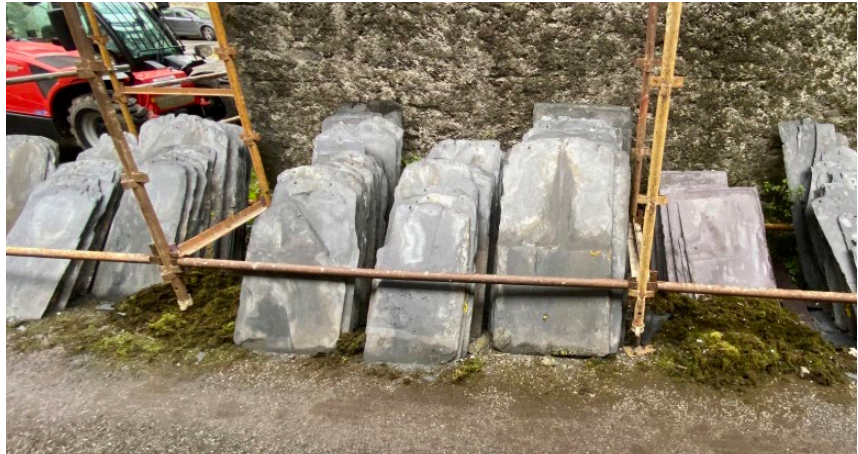
Figure 47 - Salvaged slate on site from the 2021 works - reinstated on the roof
