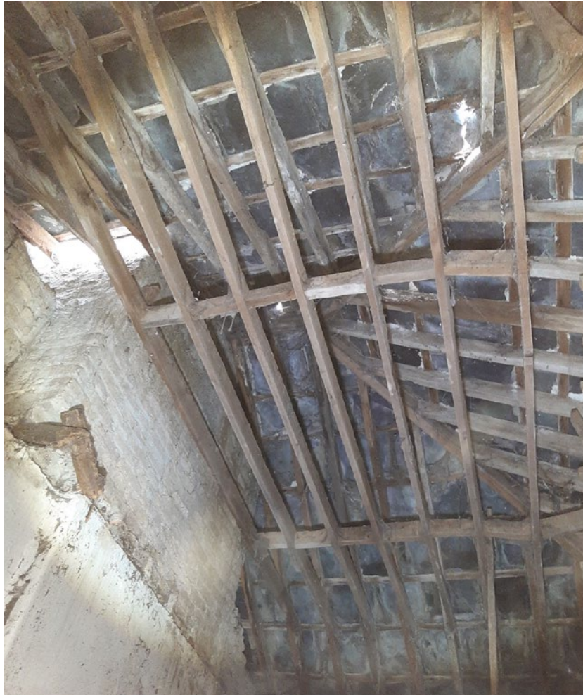
Figure 23 - Underside of roof prior to works in 2021
