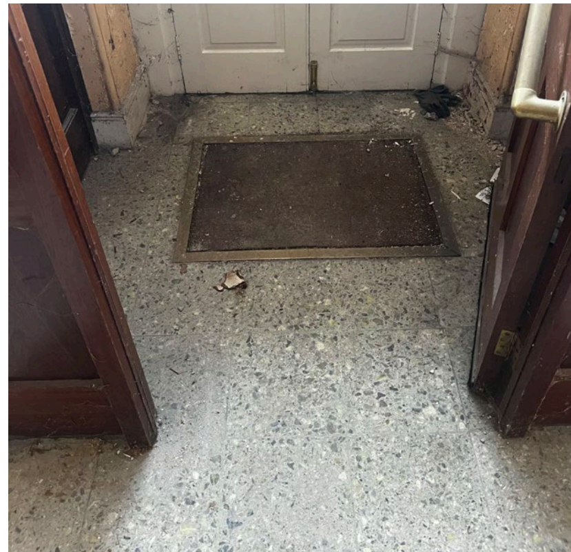
Figure 28 - Modern raised floor in the entrance hall
