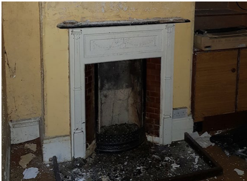
Figure 37 - Cast Edwardian fireplace in rear extension
