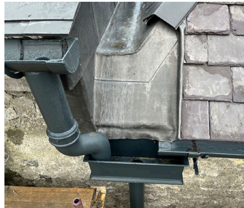
Figure 14 - Renewed rainwater goods to rear of building (completed in 2021)
