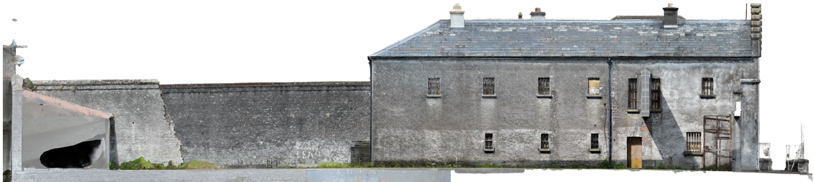
Figure 41 - Rectified photographic view of the south facade
