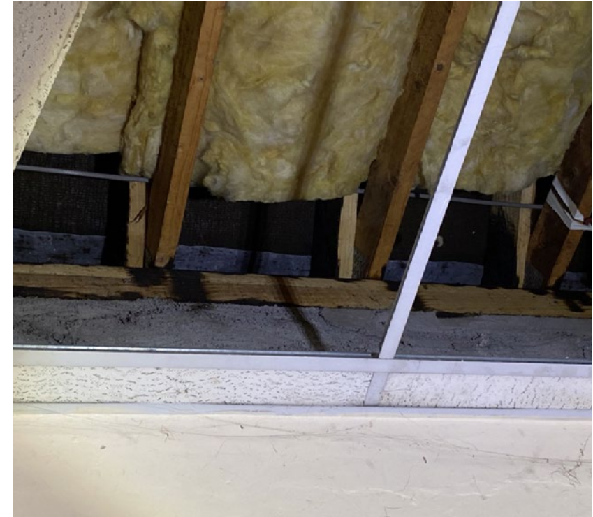
Figure 24 - Modern roof and ceiling above the courtroom
