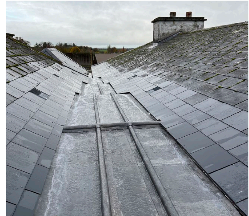
Figure 15 - Leadwork valleys repaired and fully renewed in 2021
