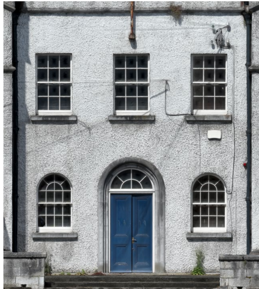
Figure 20 - Front facade entrance door and surrounding windows (repaired 2021)
