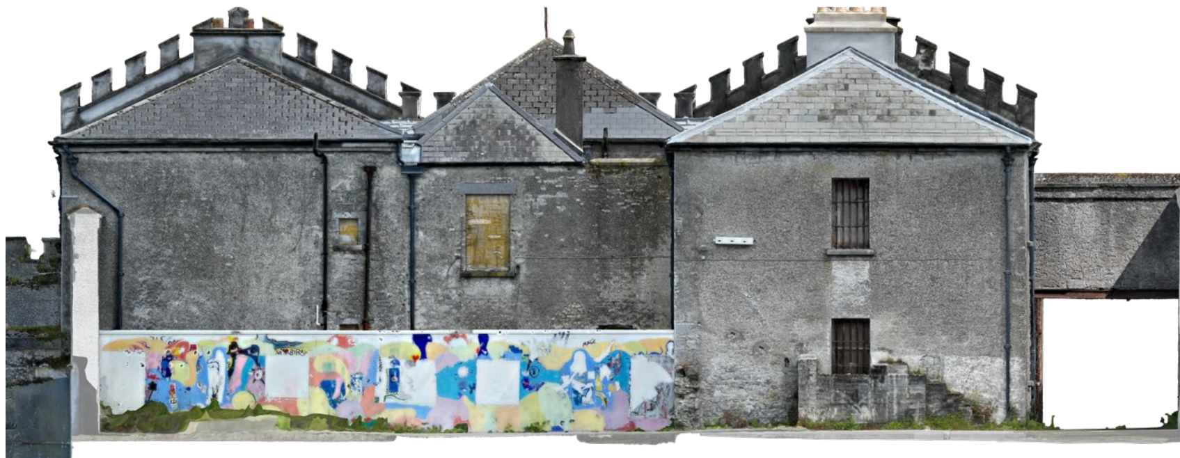
Figure 16 - Rectified photographic view of the rear facade of Birr Courthouse
