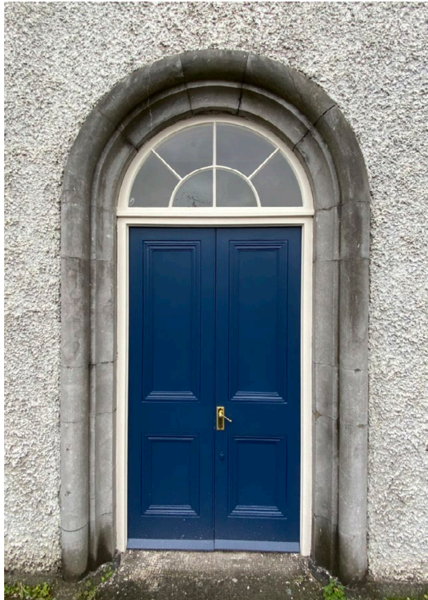
Figure 11 - Front Door, repaired in 2021
