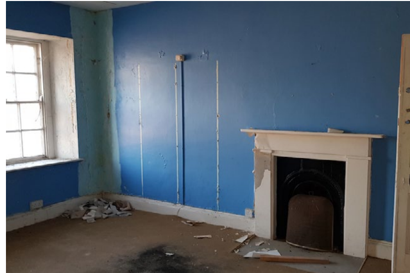
Figure 34 - Painted Victorian fireplace in first floor room in the central range
