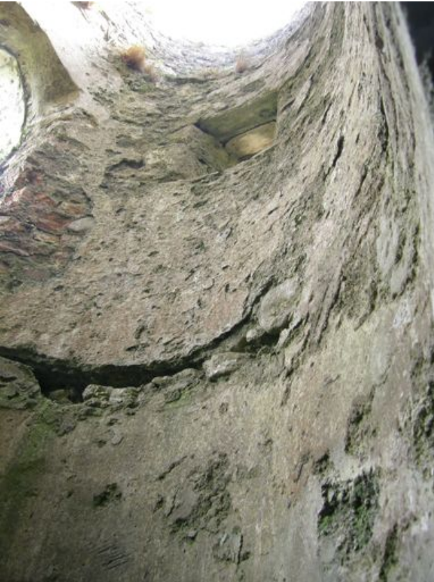
22 Inner drum looking upward to roof ledge
