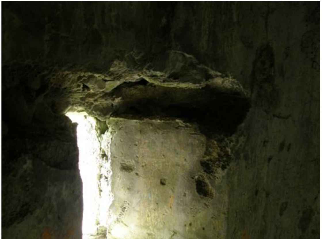
24 Loop showing socket for timber lintol
