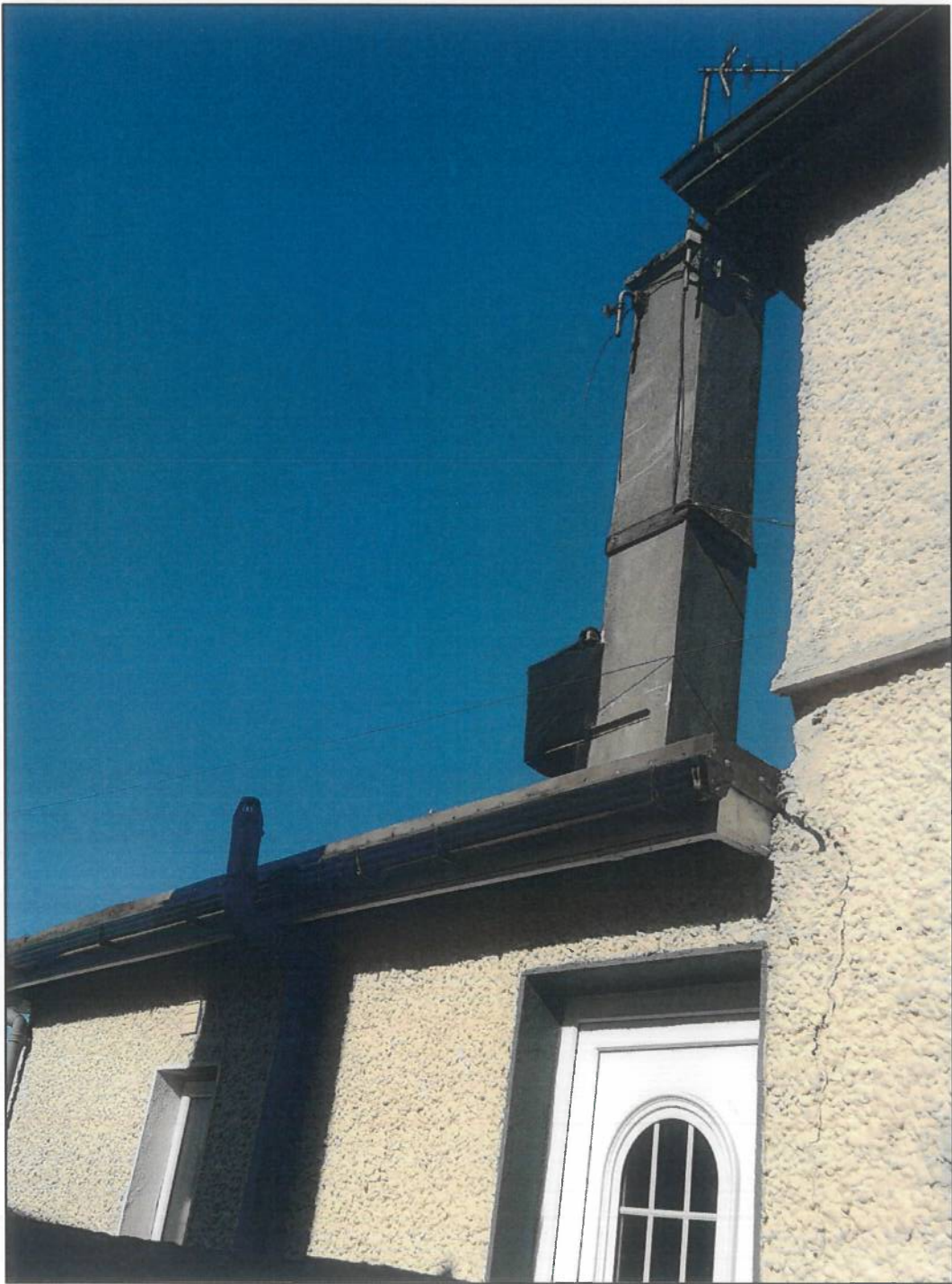
Photo 1: Rear flat-roofed kitchen extension with chimney to be removed
