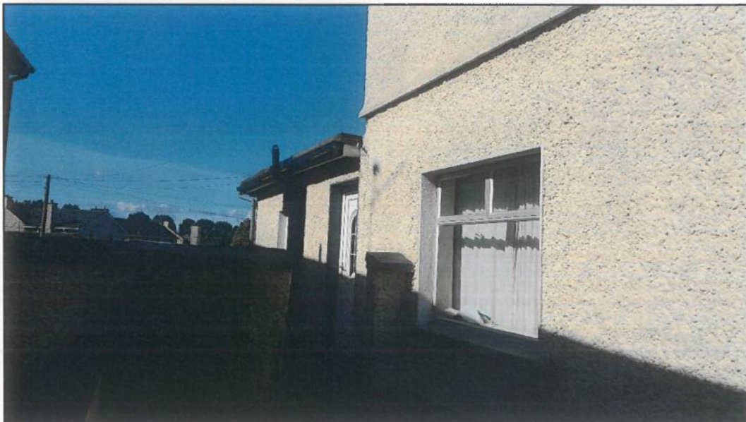
Photo 3: Side view of rear flat-roofed extension
