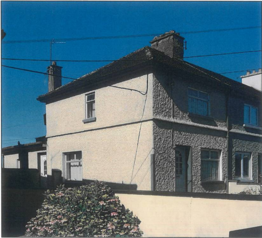
Photo 2: Existing dwelling with flat-roofed extension to the rear
