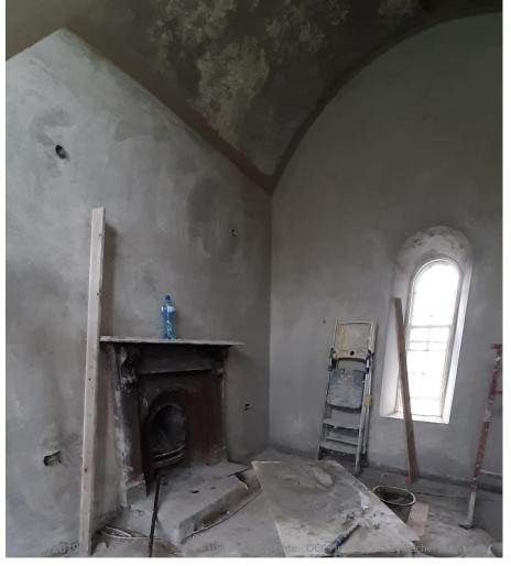
A steel flue has been installed and the chimney cleared ensuring a viable fireplace in the main central room.
