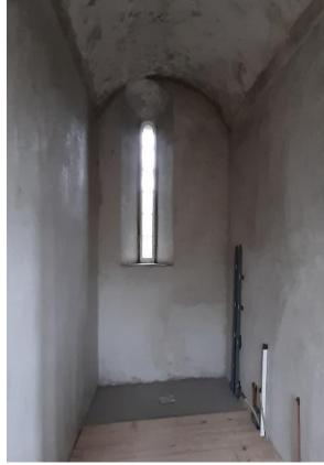
Before + After –Walls: lime plaster and timber floors
