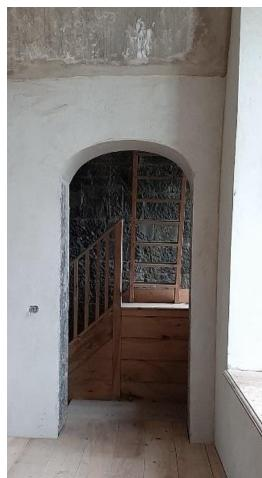
Before + After –Walls: lime plaster and timber floors
