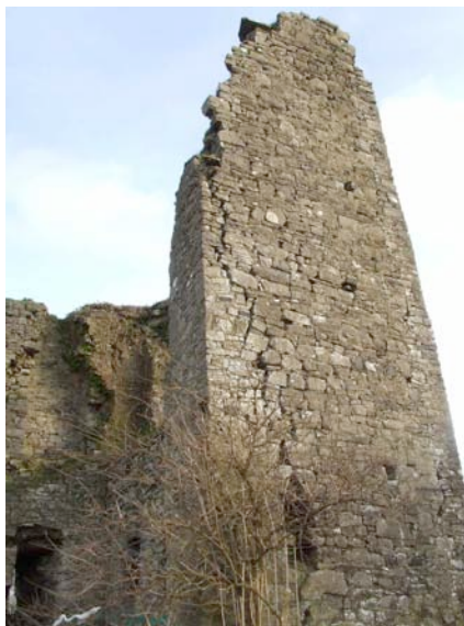
S end of W wall, from W
