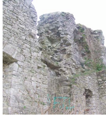
E wall ground floor, first floor, from NW
