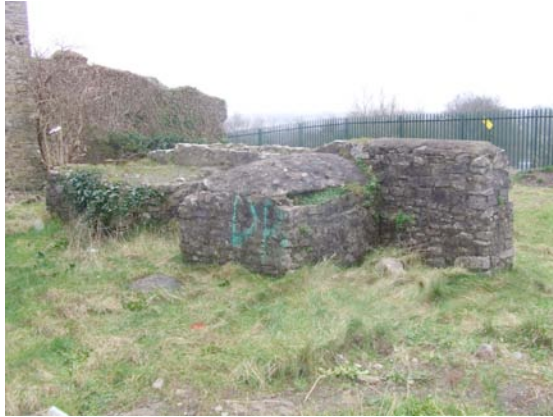
Early masonry stump and embrasure, W wall, from NE
