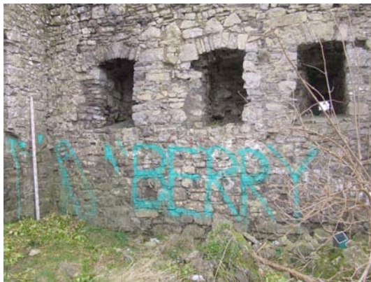
Lengthened aumbries and shortened loop, S wall inside
