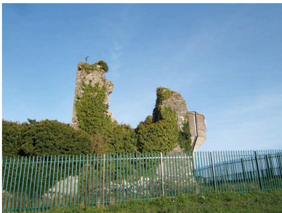
Palisade fencing and water tower in background would benefit from screen planting
