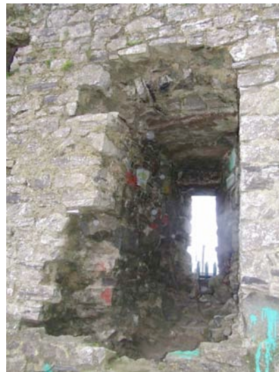
Slabs and wicker centring, roof of E wall loop, from W.
