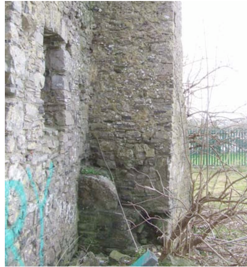
Early masonry stump, SW corner, from E.
