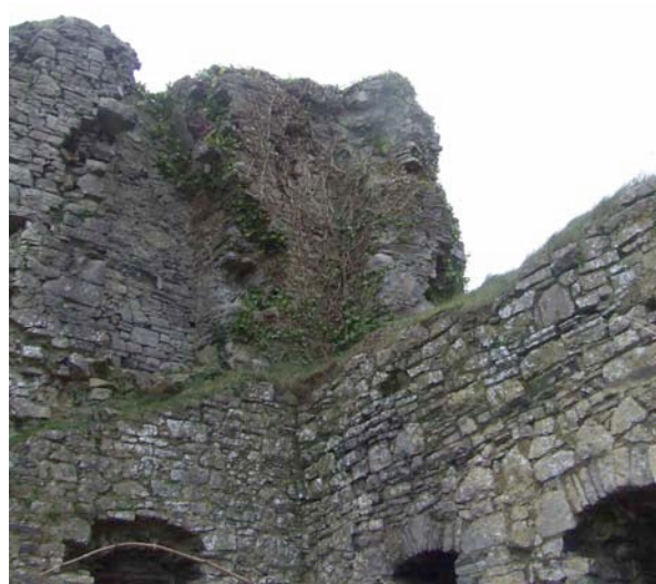
Blocked mural passage/ stair, SE corner, from NW.
