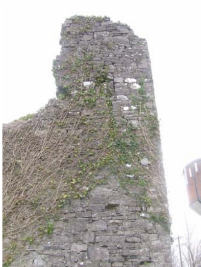
Blocked light, first floor, SE corner, from S.
