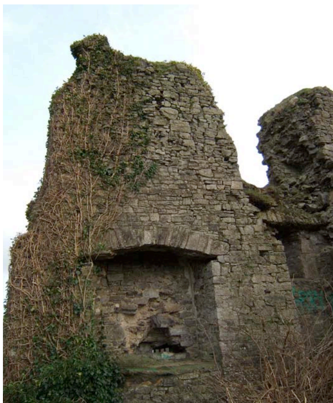
Condition of masonry inner face of east wall
