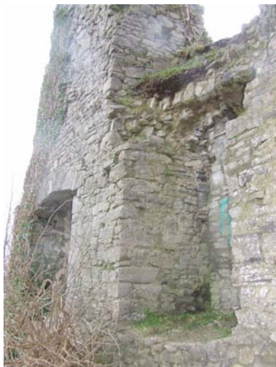
E wall, inserted fireplace and central embrasure, ground floor, from SW.
