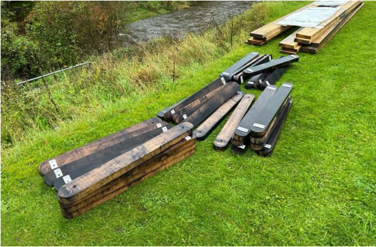
Deck Ready for Installation
