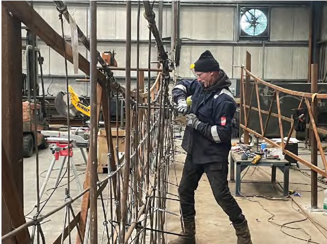
Checking and Retying all Connections
