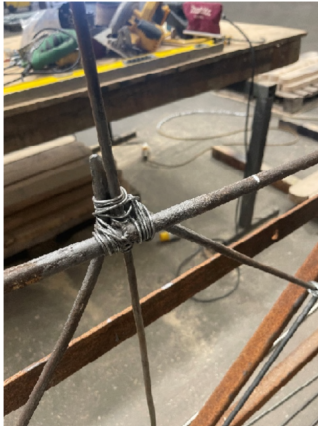
Wire Connection Detail
