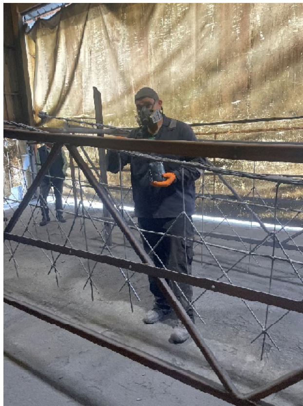
Micaceous Oxide Coating
