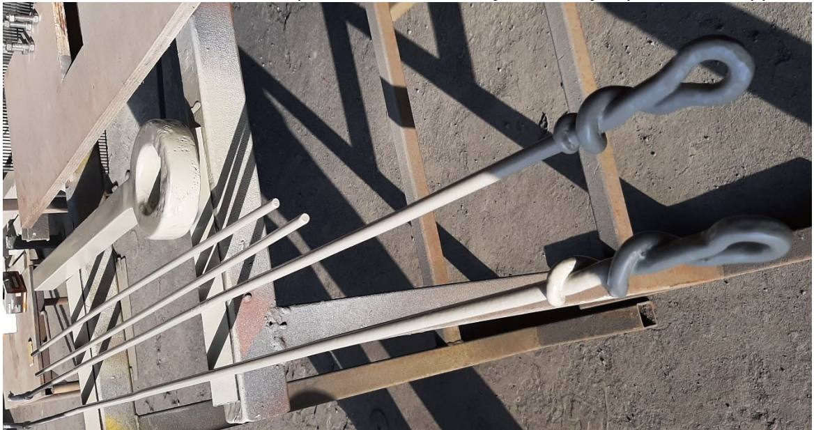
Circular-ended connector with replacement extension, first coat of 12y undercoat applied
