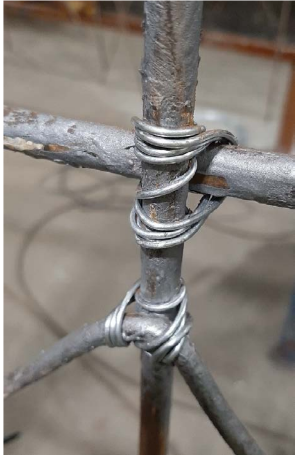
Repairs underway, new binding wire to strengthen structure
