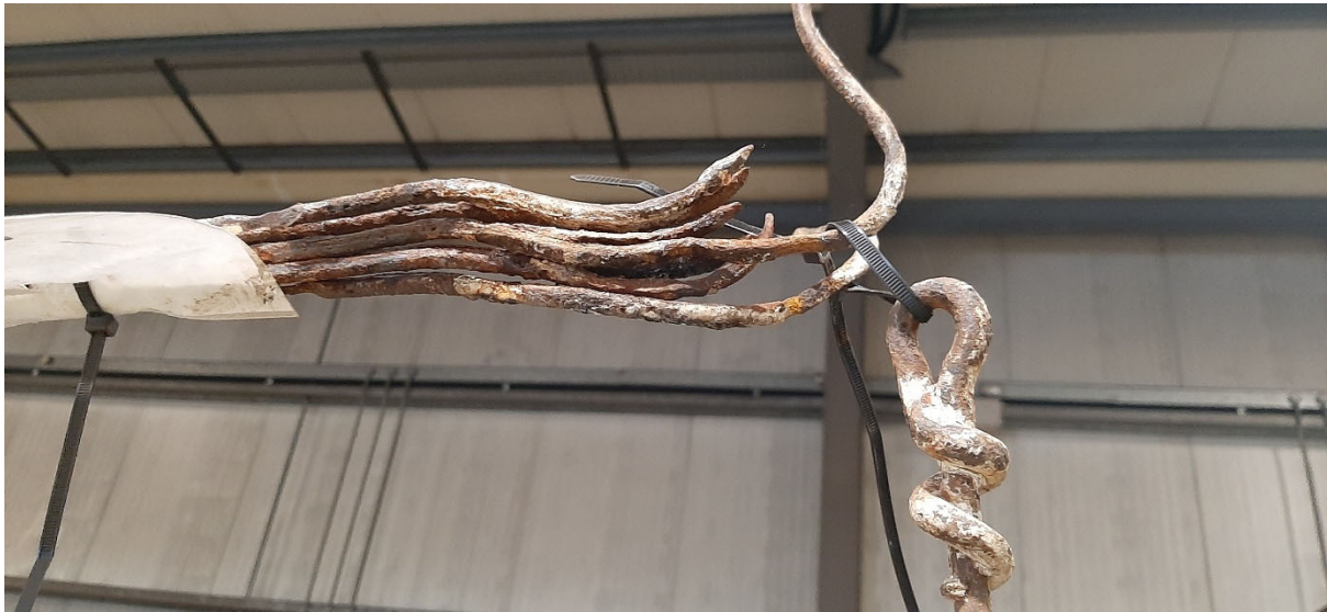
Top chord multi-strand – connecting detail required, proposed below
