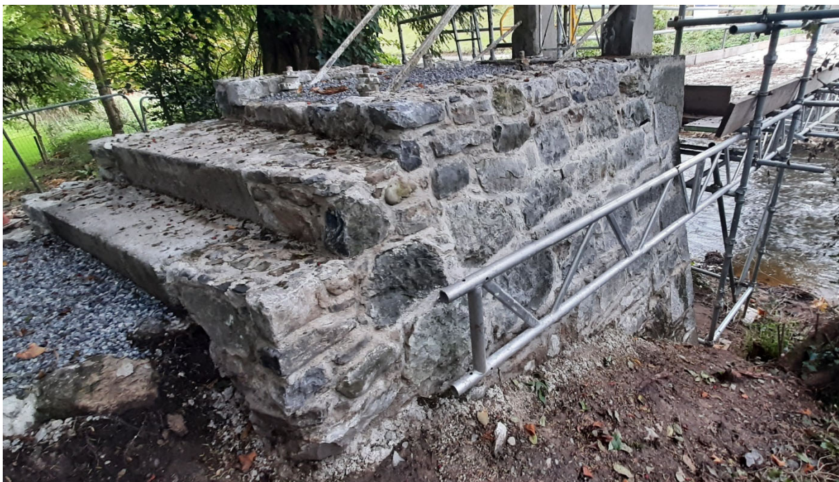
Existing stepped approach repaired
