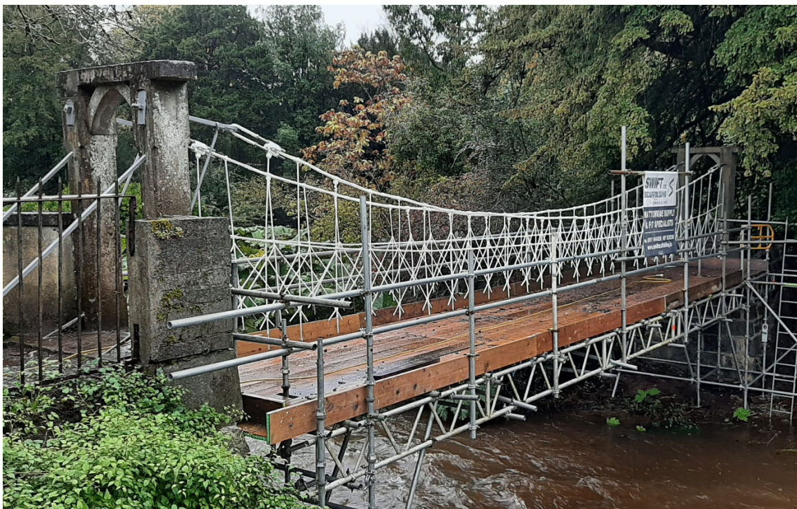
Sides in place and fixed to supports – awaiting timbers
