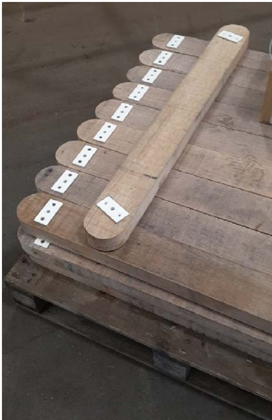
2023_0926 timber deck cross-timbers with underside fitting to allow for movement and timber decking prepared – all timbers from Birr estate
