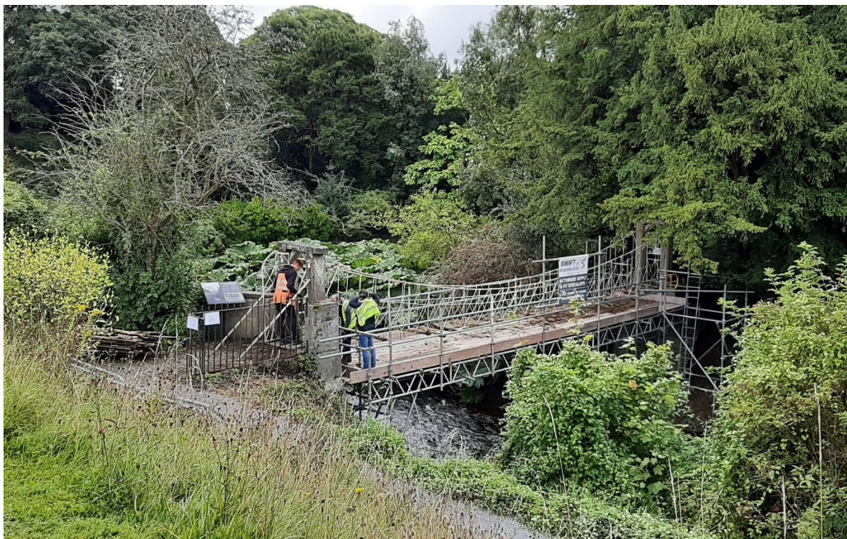
Bridge removed from site to Mackey's 2023_0828
