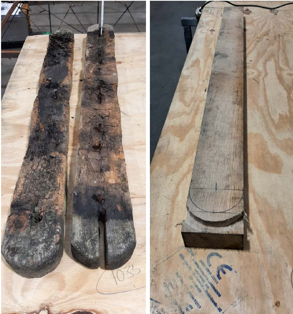
Existing timber deck cross-timbers used as replica for replacement sections
