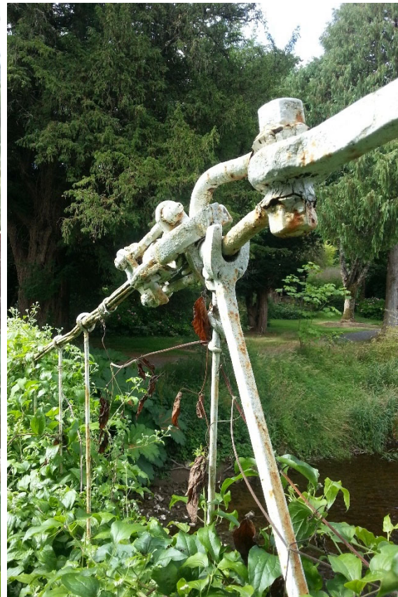
Fixing details – repairs over time. Note circular-ended connector, later repaired in Mackey’s
