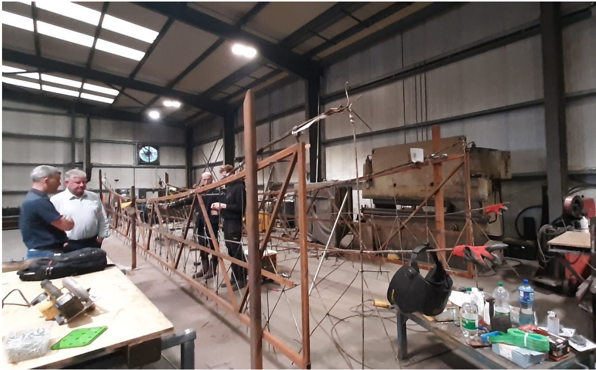
Both sides of suspension bridge, hanging on custom frame at Mackey's 2023_0911
