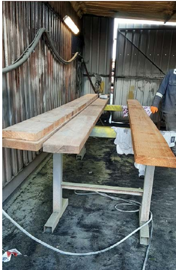
2023_0926 timber deck cross-timbers with underside fitting to allow for movement and timber decking prepared – all timbers from Birr estate
