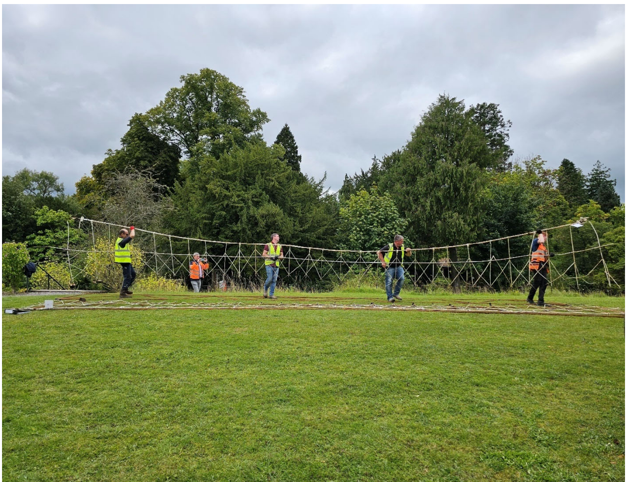
Bridge removed for setting on custom frame (frame also used in workshop)
