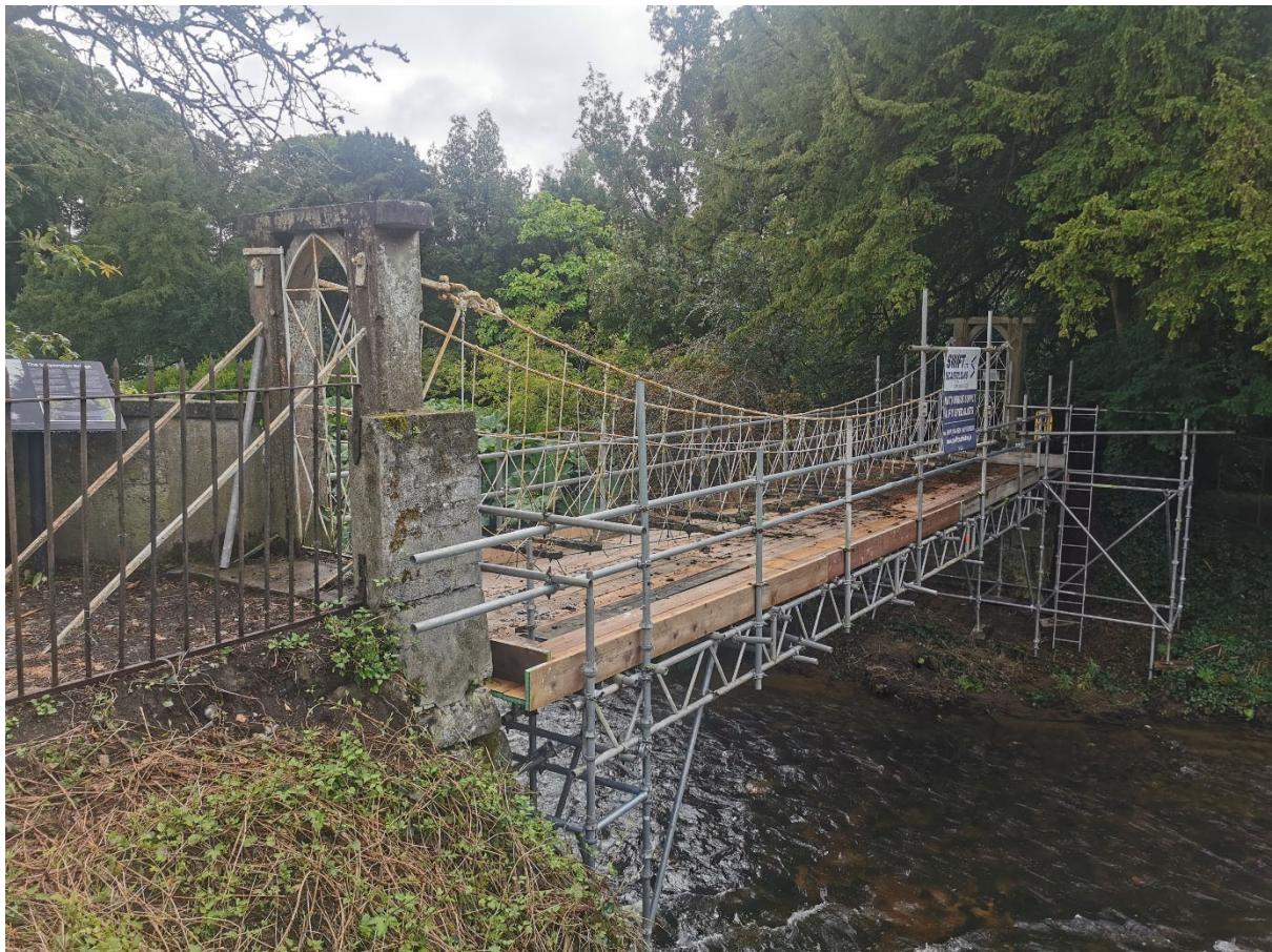
Scaffolding erected for bridge removal
