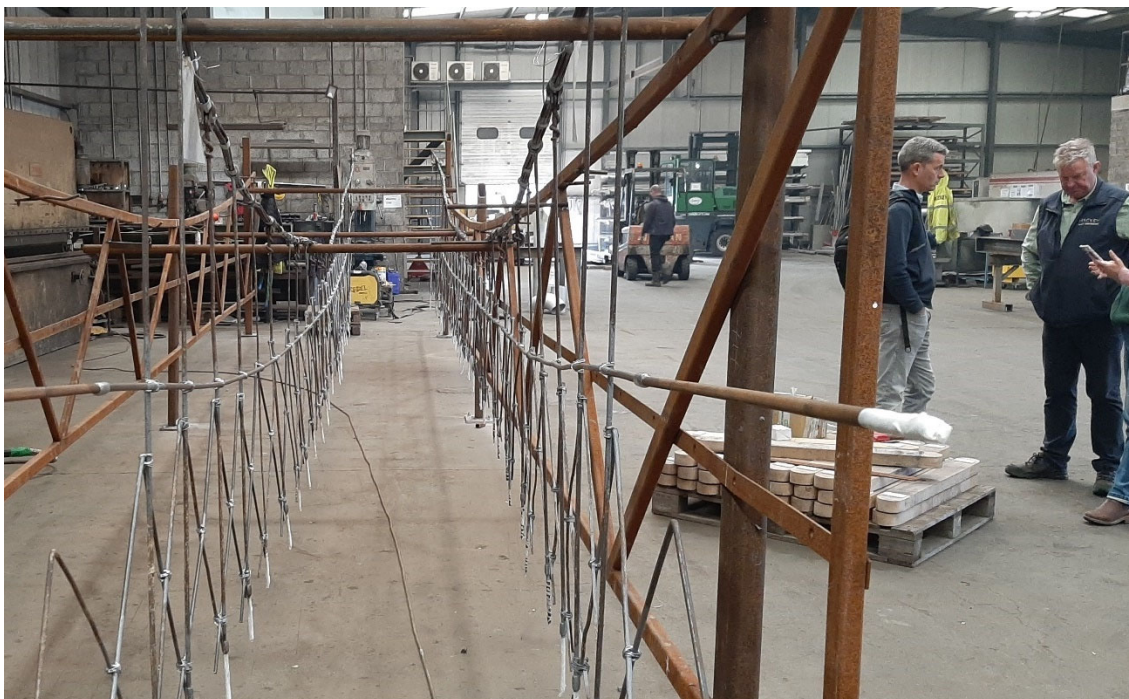
Frame considerably strengthened with binding throughout
