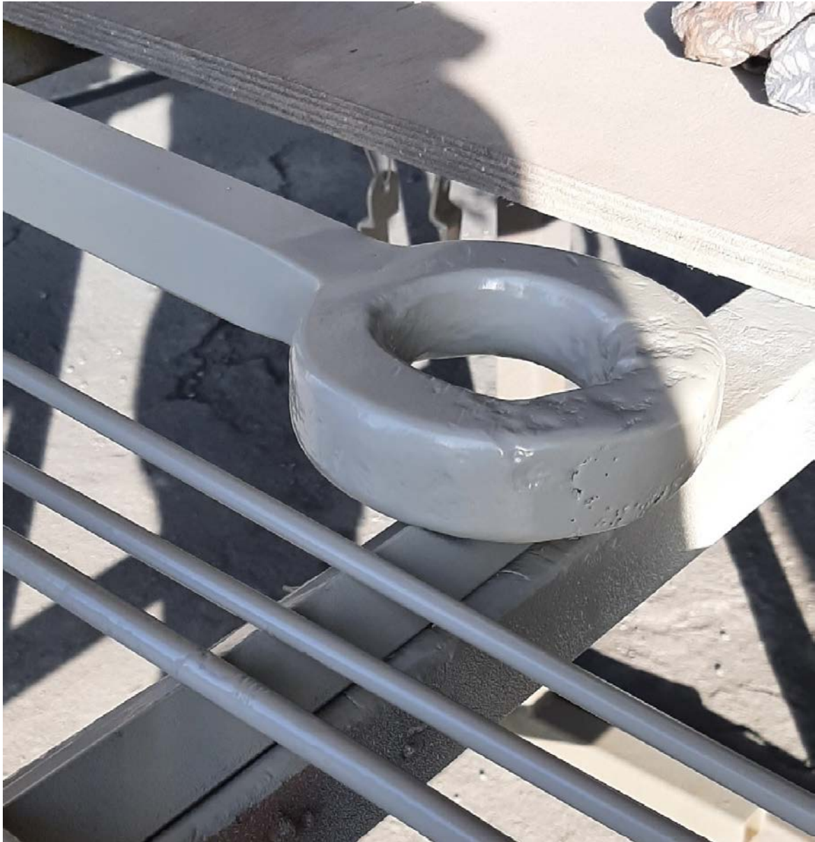
Circular-ended connector with replacement extension, first coat of 12y undercoat applied
