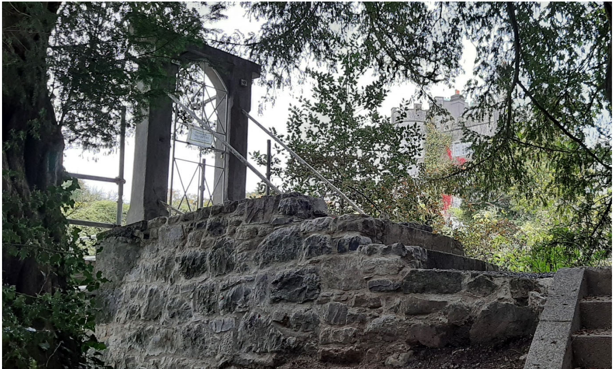
Raised embankment to far bank
