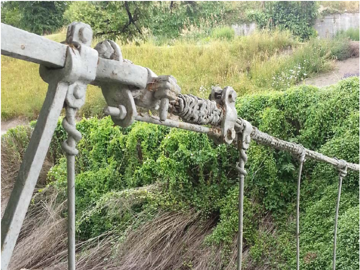
Fixing details – repairs over time. Note circular-ended connector, later repaired in Mackey’s
