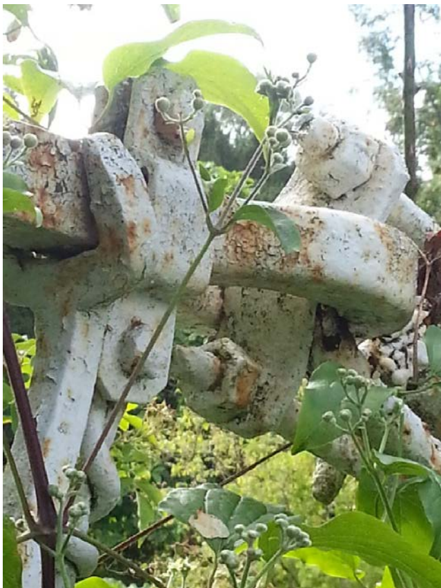
Fixing details – repairs over time. Note circular-ended connector, later repaired in Mackey’s
