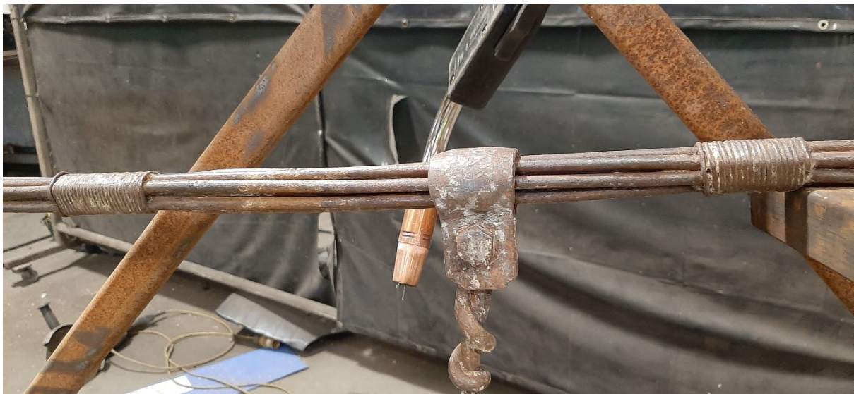
Existing binding retained where sound
